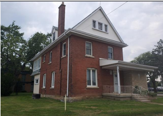
8. East side window (note aluminum frame, stone sill and voussoirs)
