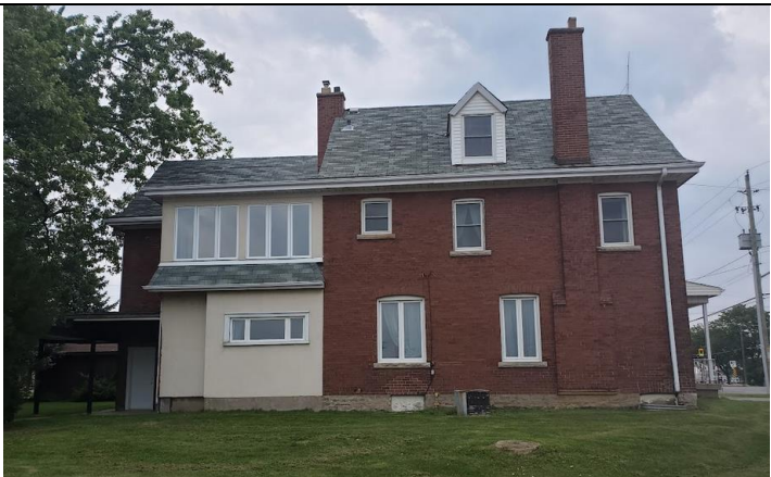
7. West side door from 1920 renovation (note difference in masonry)
