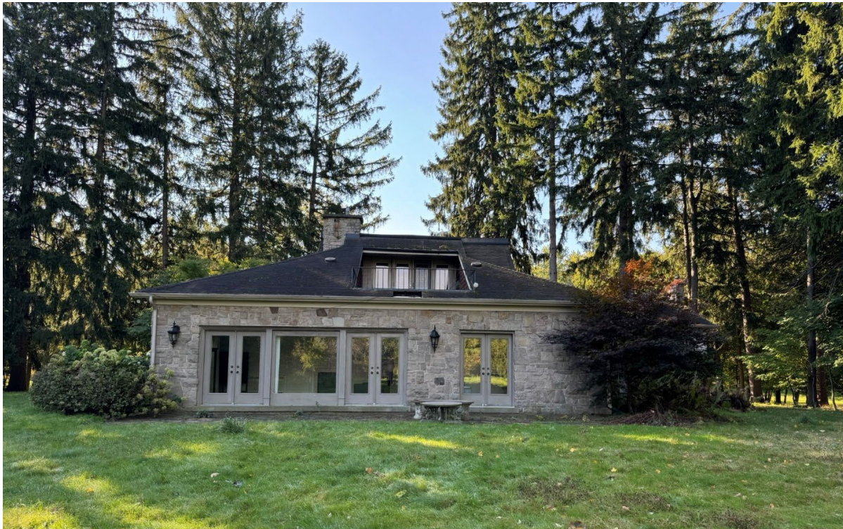
Figure 13: North (Rear) Façade of 163 Sulphur Springs Road
