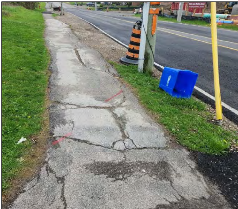
Figure 2.3) West 5 th Street Sidewalk Condition – Heavy Vehicle Damage
