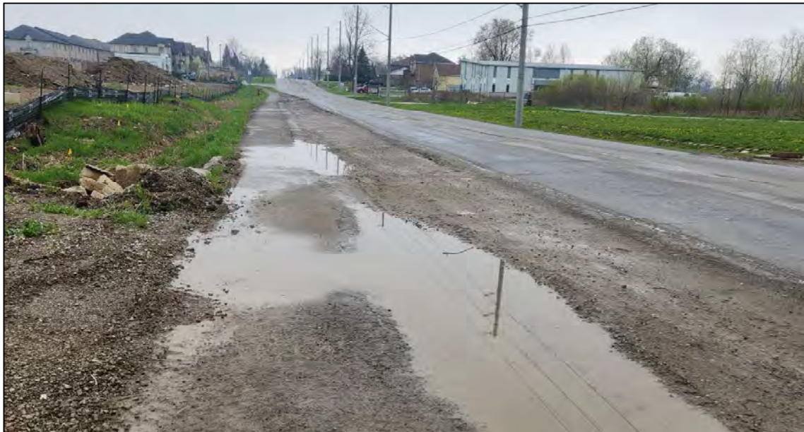
Figure 2.1) West 5 th Street Sidewalk Condition – Drainage
