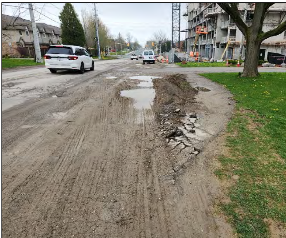
Figure 2.3) West 5 th Street Sidewalk Condition – Heavy Vehicle Damage
