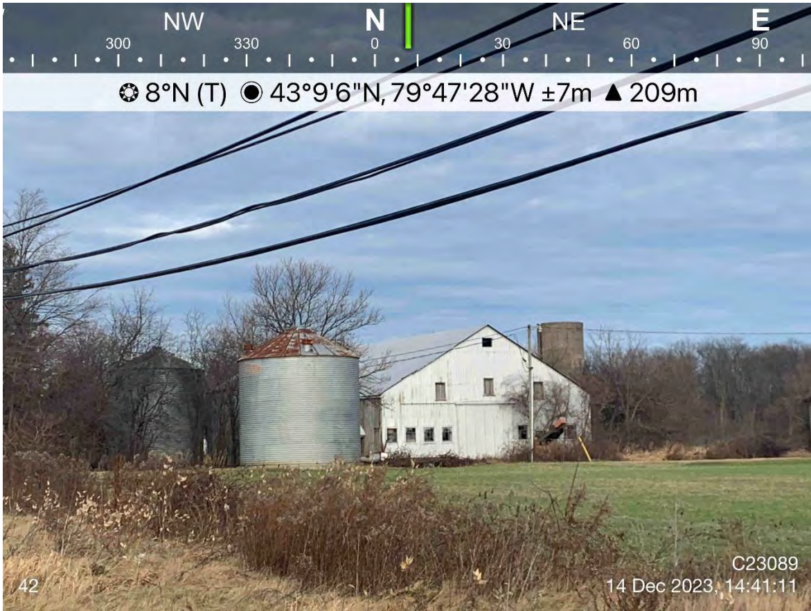
Photo 7: Operation #42 – Unoccupied Livestock Facility showing barn, uncapped silo, and grain bins.
