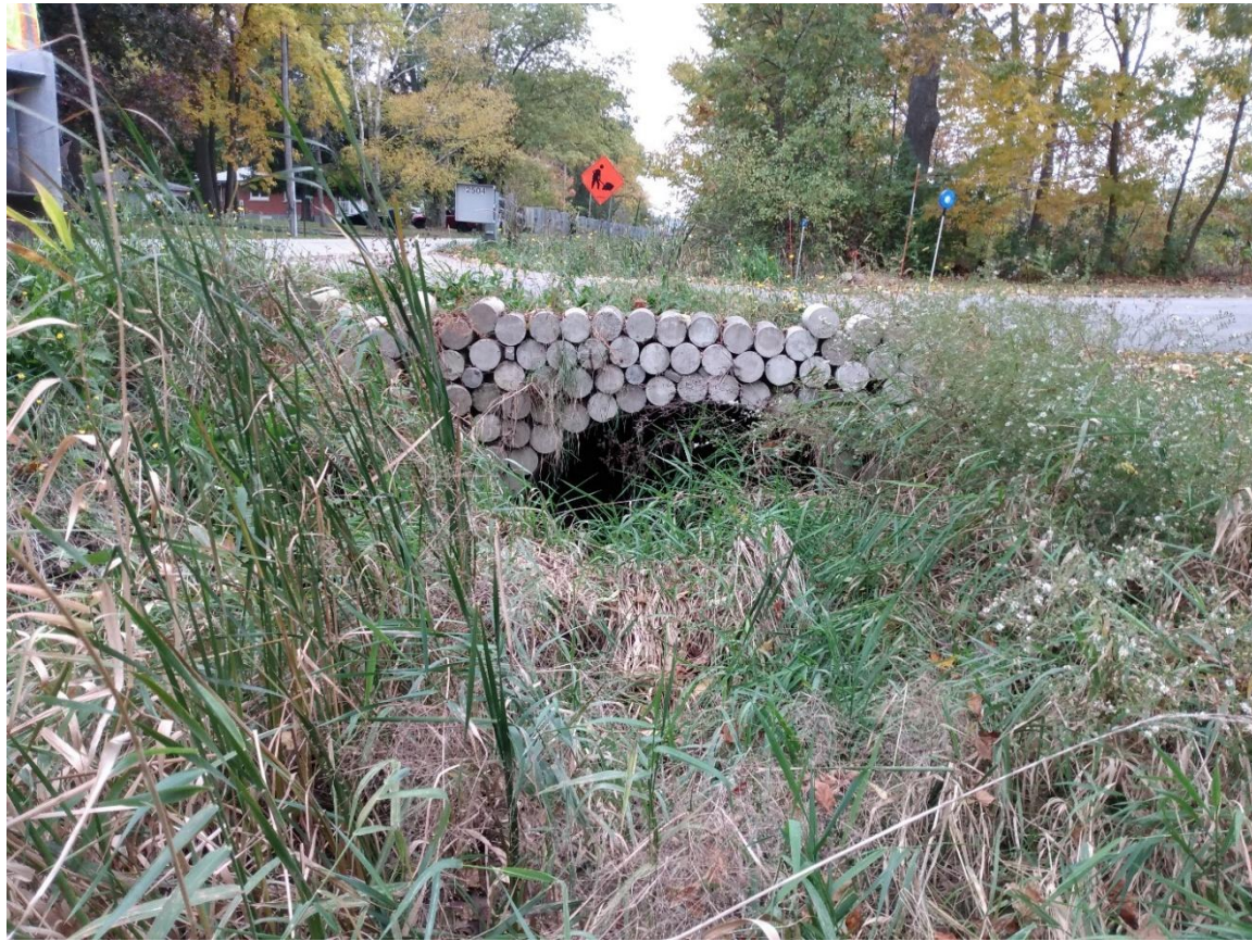
Culvert connecting Golf Club Road to a private residence near downstream end of reach.
