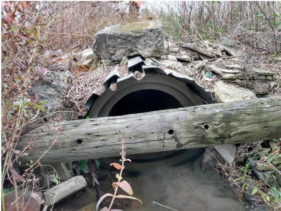
Upstream face of culvert
