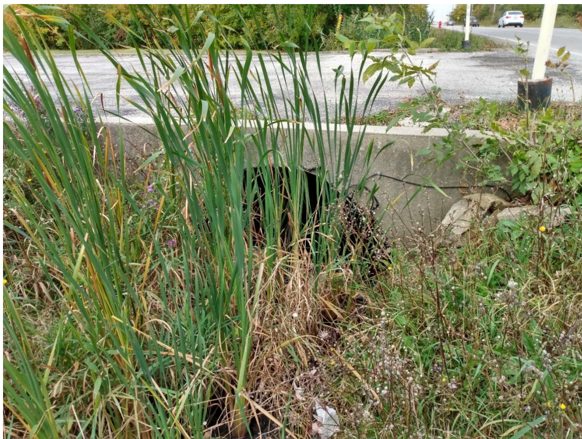
Concrete culvert connecting Mud Street East to private residence (facing downstream).
