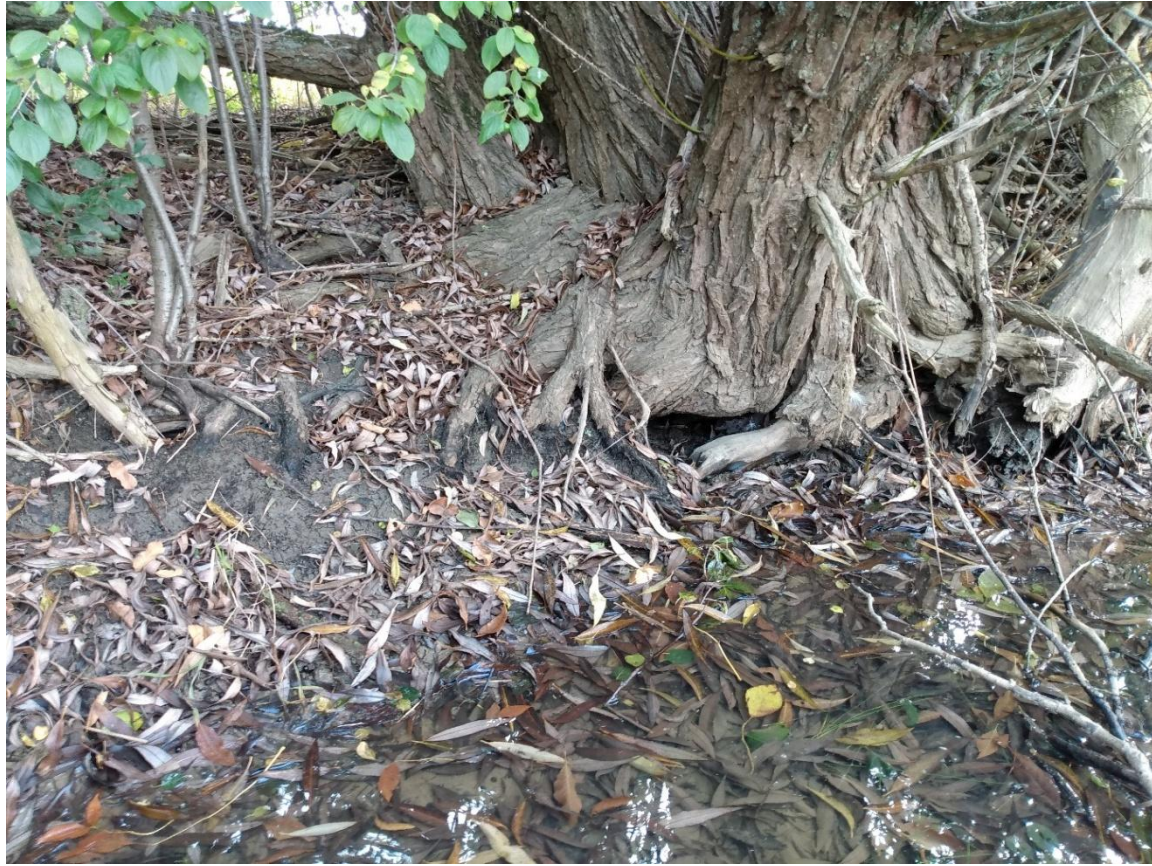
Exposed tree roots in downstream portion of the reach, indicating minor local erosion.
