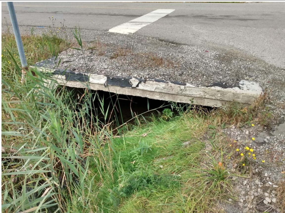
Concrete box culvert under First Road East (facing downstream).
