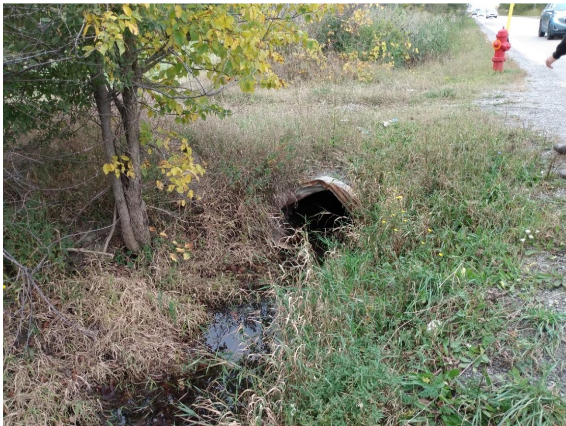
Corrugated steel culvert connecting Mud Street East to agricultural field near upstream extent of reach (facing downstream).
