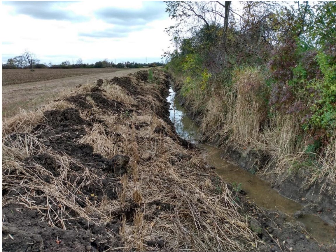
Typical view, facing upstream. Majority of reach is recently excavated.
