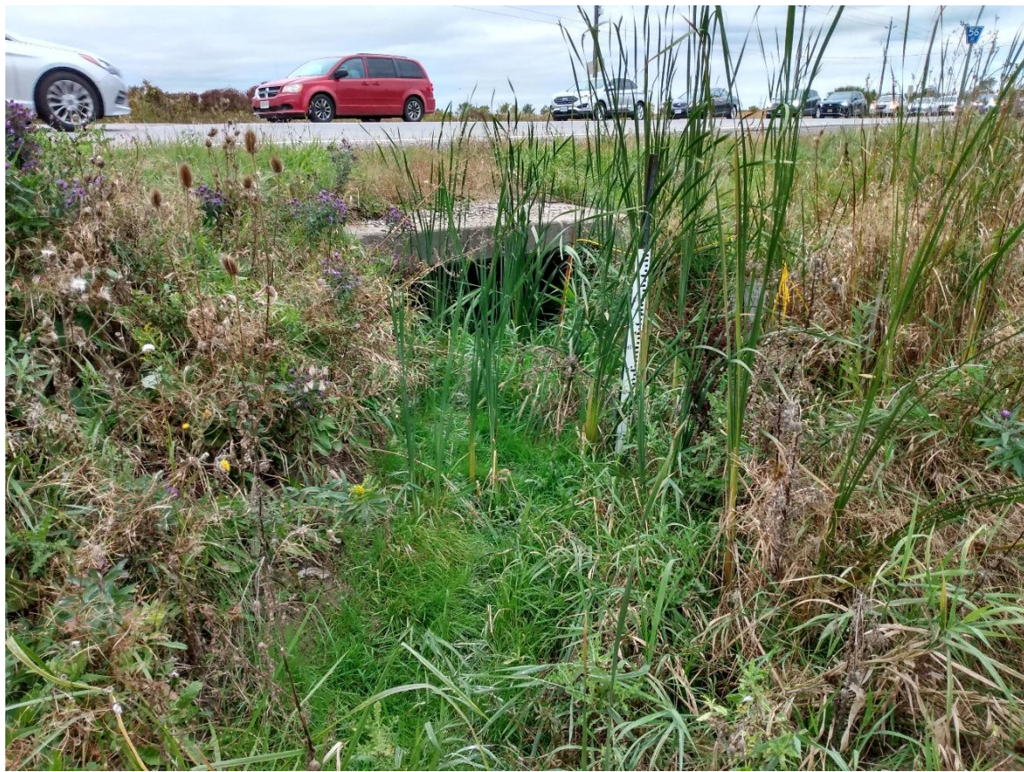
Box culvert at Highway 56 (upstream extent of reach).
