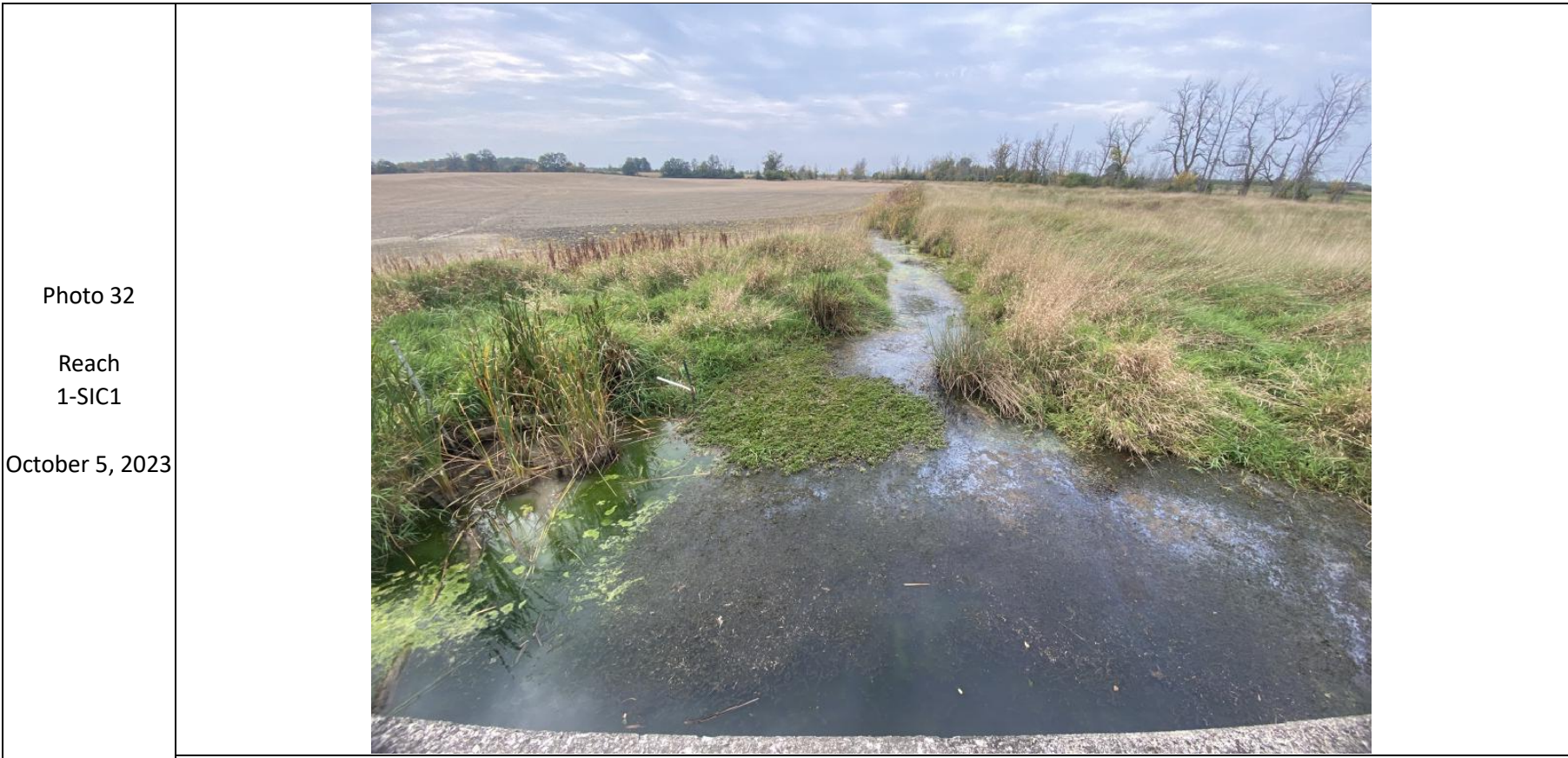
Facing upstream from the concrete box culvert at Hendershot Road.
