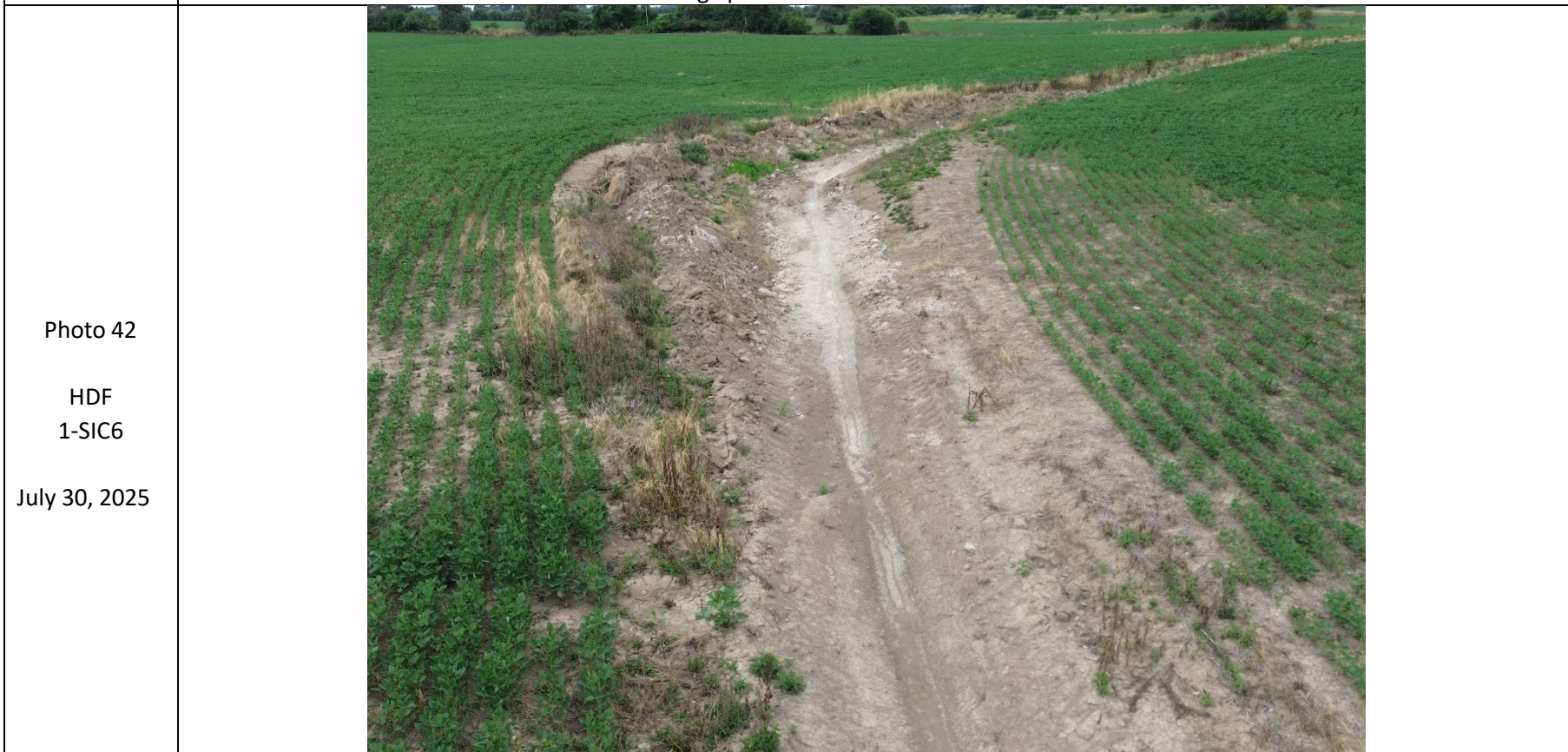
Facing upstream along HDF 1-SIC6 during dry conditions. Additional piled unconsolidated sediments and tracks along the HDF provide evidence of recent modifications.
