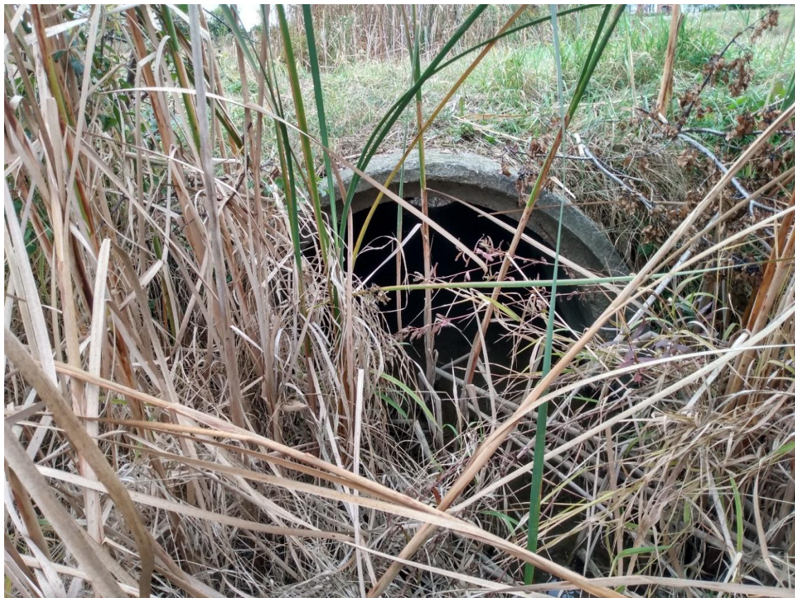
Concrete culvert connecting agricultural fields (facing upstream).
