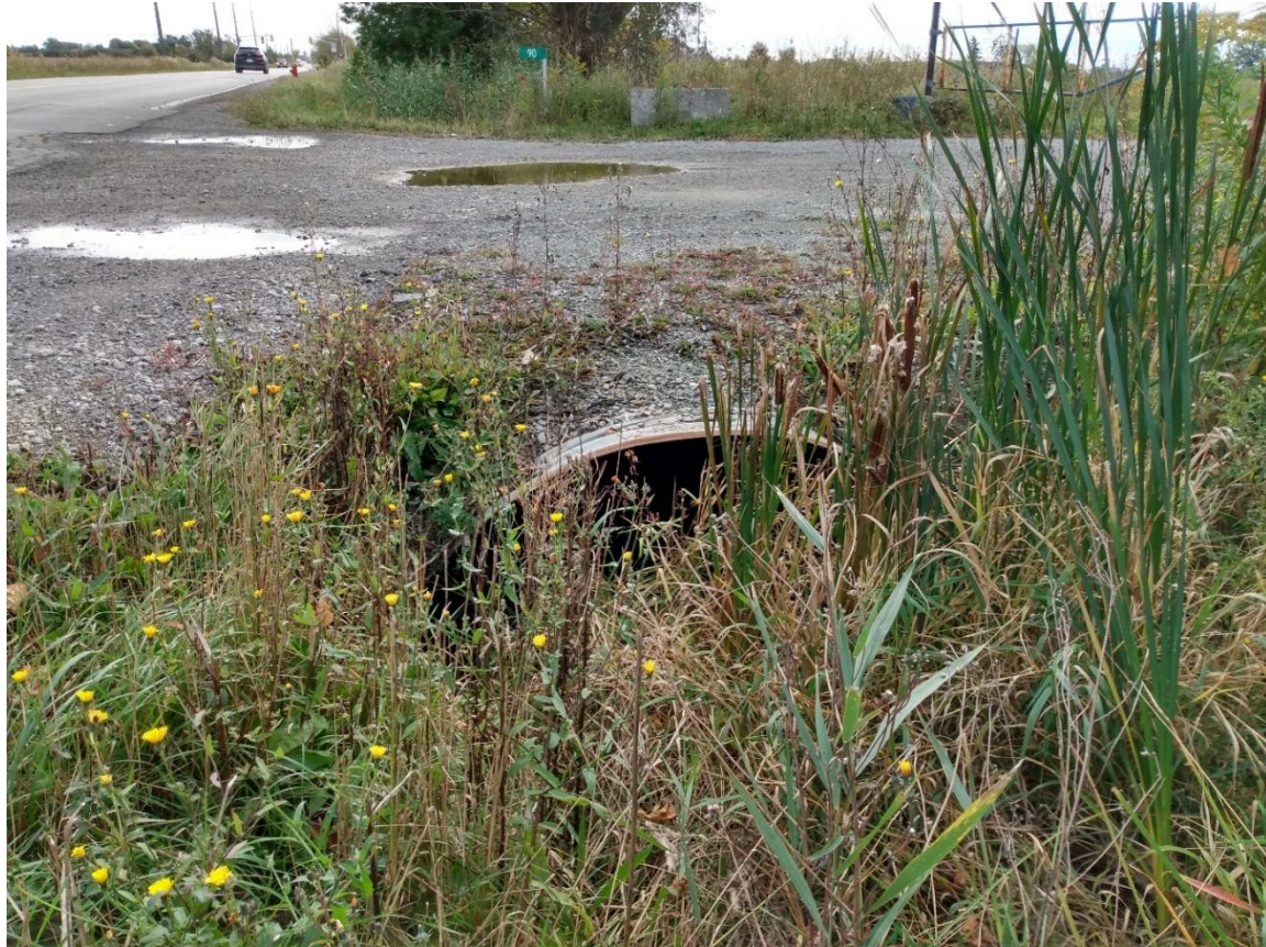
Corrugated steel culvert connecting Mud Street East to private residence (facing upstream).
