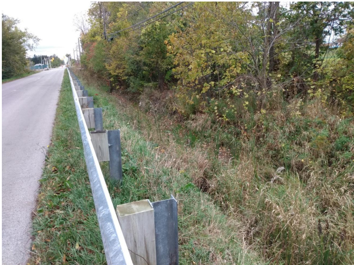
Typical section of reach. Roadside ditch bordering agricultural fields.
