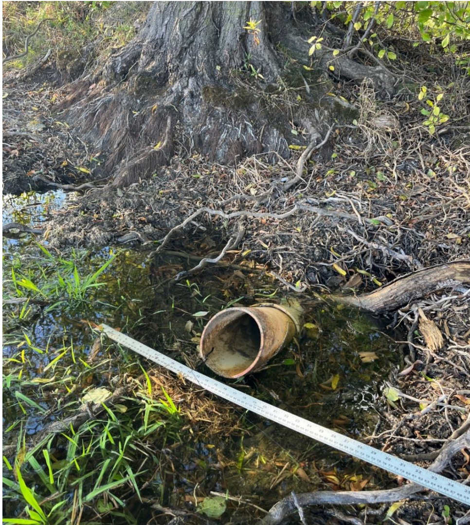
Photo 44: 3-SC1 Pond (October 23, 2025). Tile drain inlet connecting to pond.
