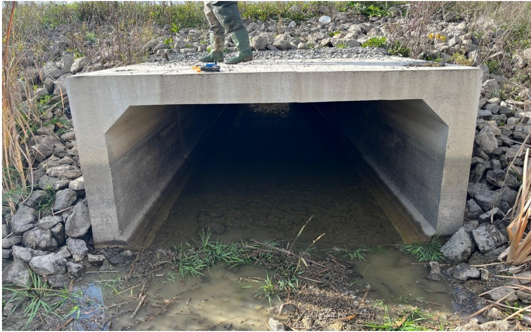
Photo 13: Reach 1-SIC5 (October 23, 2025). Outlet of crossing, facing upstream.
