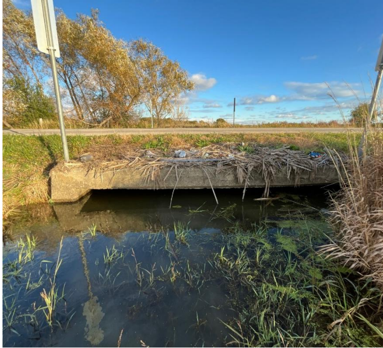
Photo 42: Reach 3-SC2 Crossing (October 23, 2025). Typical view, facing downstream.
