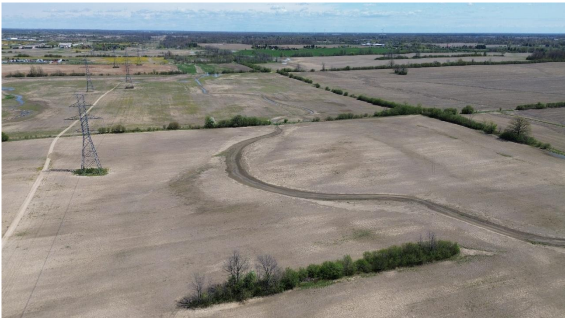
Photo 12: Reach 1-SIC4. Aerial view of channel, facing eastwards.
