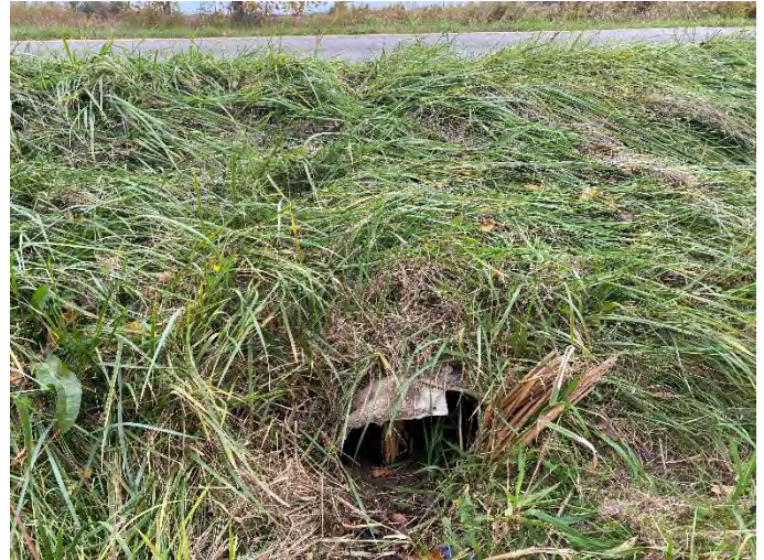
Photo 128: SHC 16 – Downstream facing upstream towards culvert.
