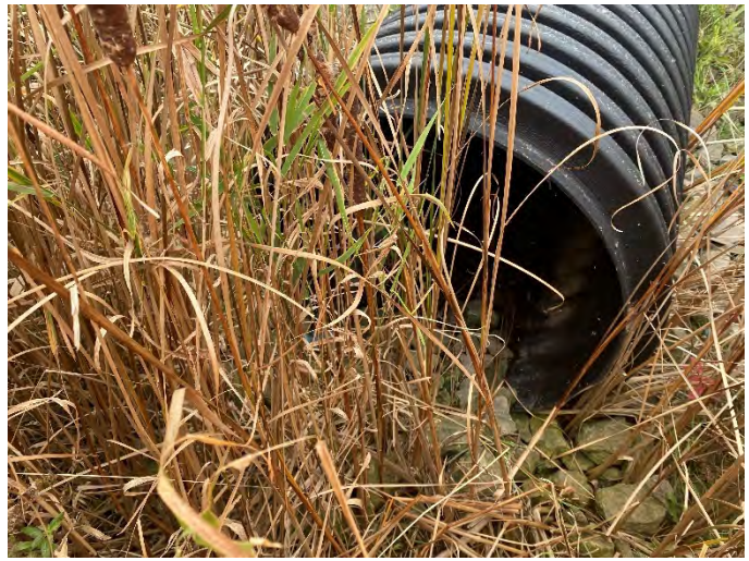
Photo 104: SHC 8 – Downstream facing upstream towards culvert.
