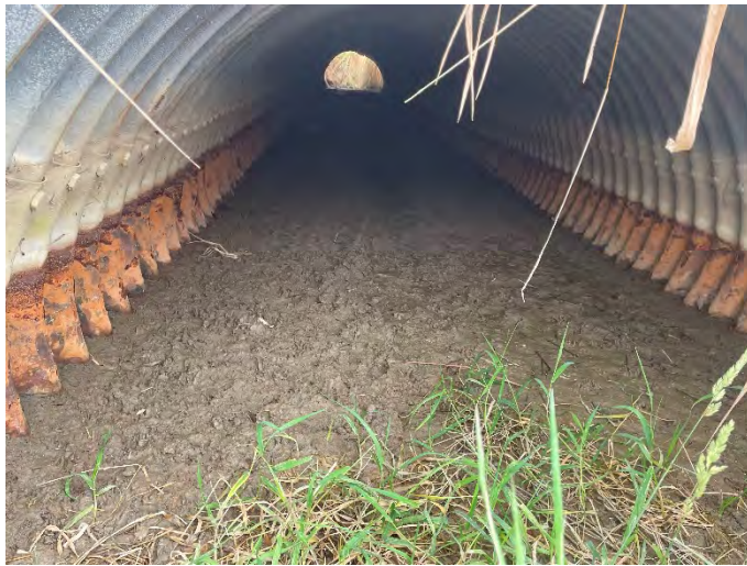
Photo 79: SHC 4 – Downstream facing upstream inside culvert.
