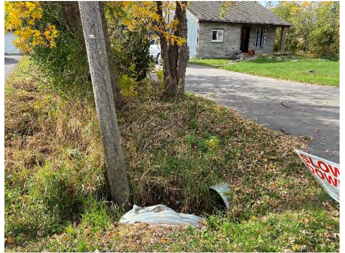
Photo 172: SC 11 – Facing upstream of culvert.
