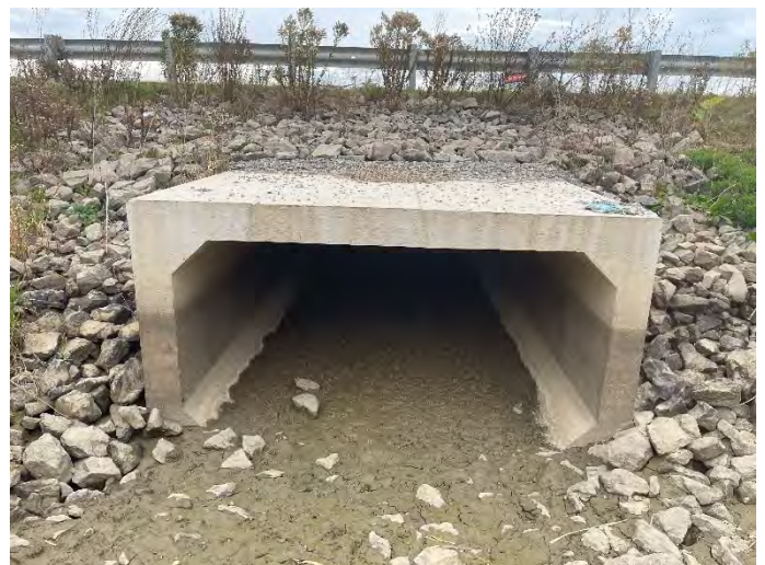
Photo 84: SHC 5 – Downstream facing upstream towards culvert.
