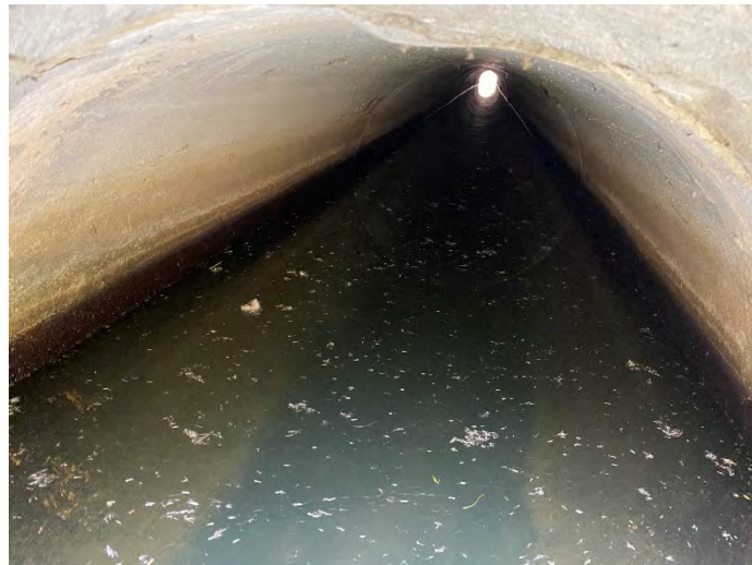
Photo 99: SHC 7 – Downstream facing upstream inside culvert.
