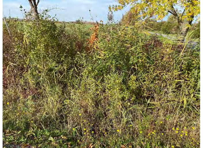
Photo 154: SC 8 – Facing upstream of culvert.
