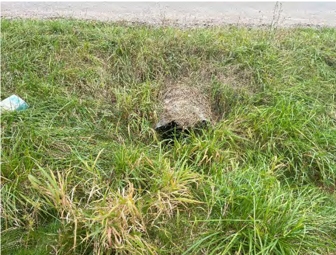
Photo 75: SHC 2 – Upstream facing downstream towards culvert.
