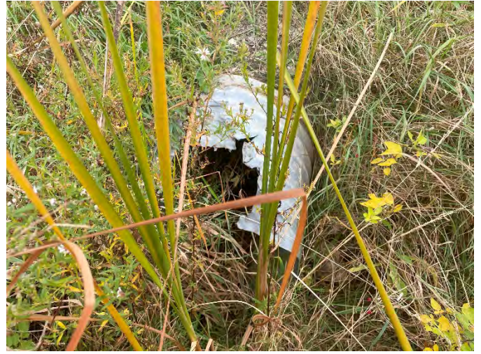
Photo 16: 20MC-W 1 – Upstream facing downstream towards culvert.
