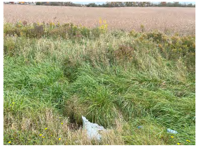
Photo 68: HC 2 – Facing upstream of culvert.
