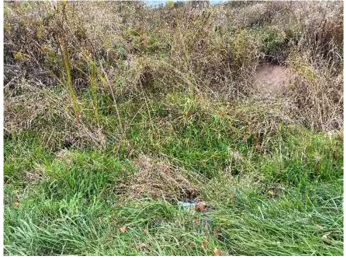
Photo 124: SHC 15 – Facing upstream of culvert.
