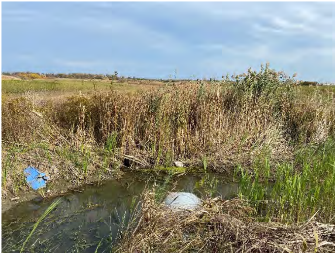
Photo 175: SC 12 – Facing downstream of culvert.
