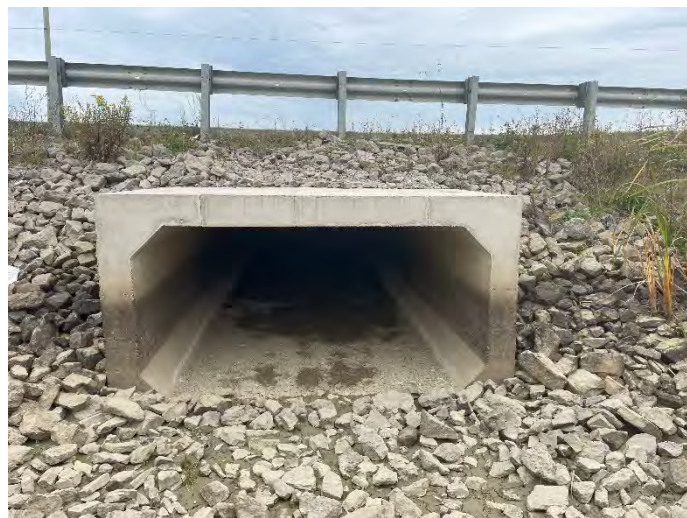
Photo 87: SHC 5 – Upstream facing downstream towards culvert.
