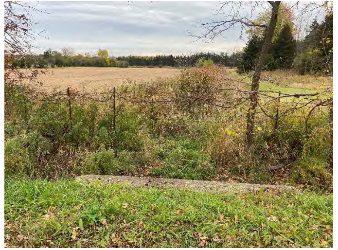
Photo 42: 20MC-E 9 – Facing downstream of culvert.
