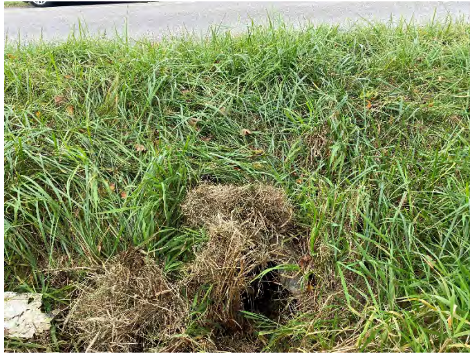
Photo 131: SHC 16 – Upstream facing downstream towards culvert.
