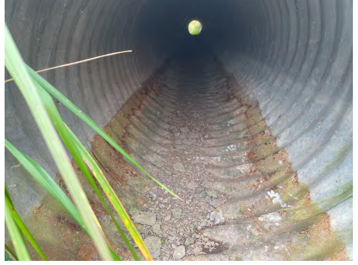
Photo 26: 20MC-W 3 – Downstream facing upstream inside culvert.
