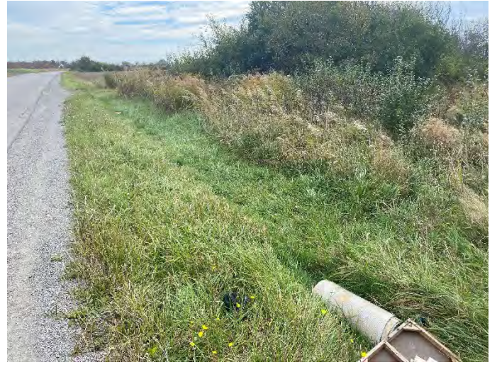
Photo 192: SC 18 – Facing upstream of culvert.
