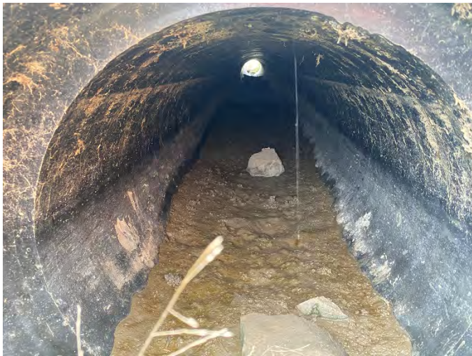
Photo 195: SC 19 – Downstream facing upstream inside culvert.
