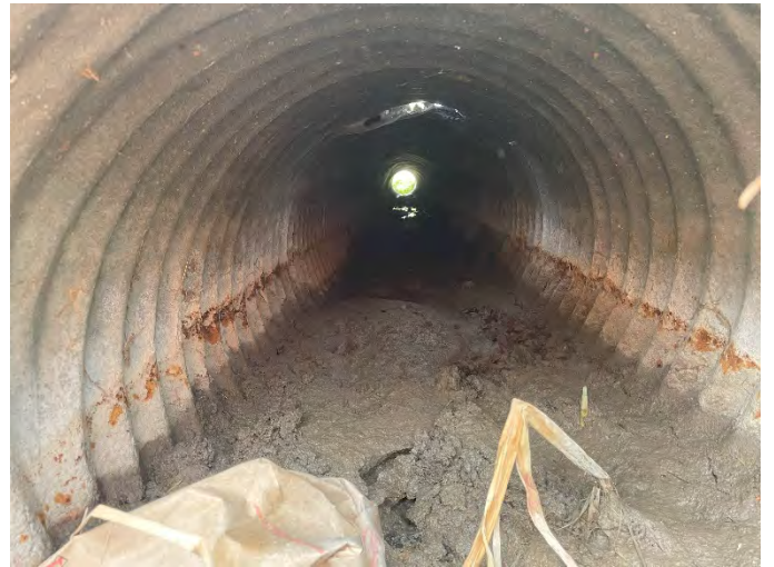
Photo 32: 20MC-W 4 – Downstream facing upstream inside culvert.
