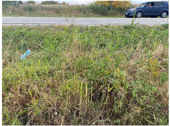
Photo 188: SC 18 – Downstream facing upstream towards culvert.
