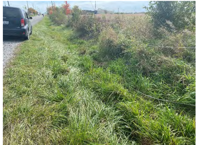
Photo 184: SC 23 – Upstream of culvert facing east.
