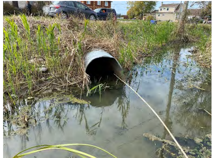
Photo 176: SC 12 – Downstream facing upstream towards culvert.
