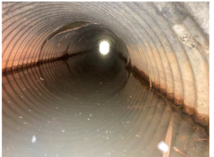
Photo 20: 20MC-W 2 – Downstream facing upstream inside culvert.
