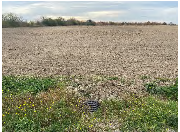
Photo 196: SC 19 – Facing upstream of culvert.
