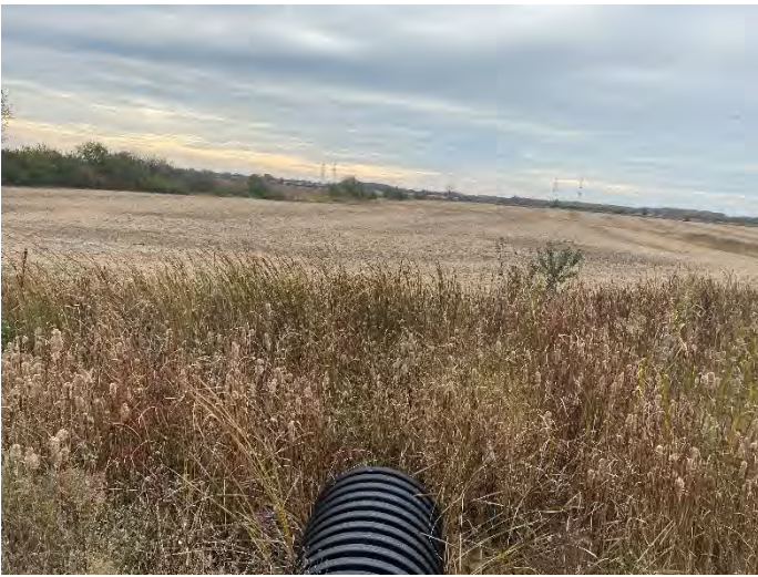
Photo 103: SHC 8 – Facing downstream of culvert.
