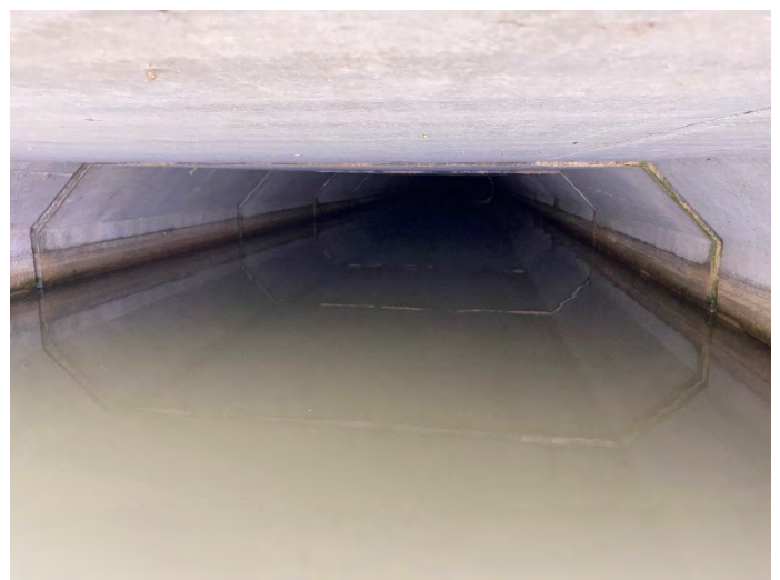
Photo 92: SHC 6 – Downstream facing upstream inside culvert.
