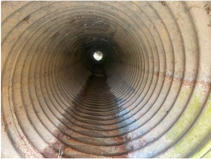
Photo 67: HC 2 – Downstream facing upstream inside culvert.
