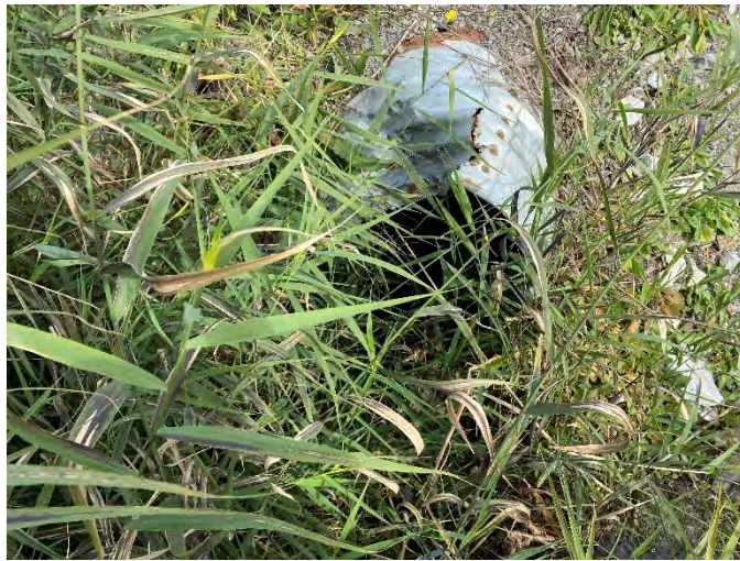
Photo 179: SC 12 – Upstream facing downstream towards culvert.
