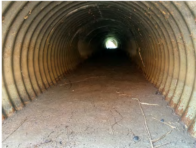
Photo 135: SHC 13 – Downstream facing upstream inside culvert.
