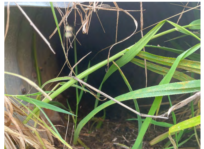
Photo 76: SHC 2 – Upstream facing downstream inside culvert.
