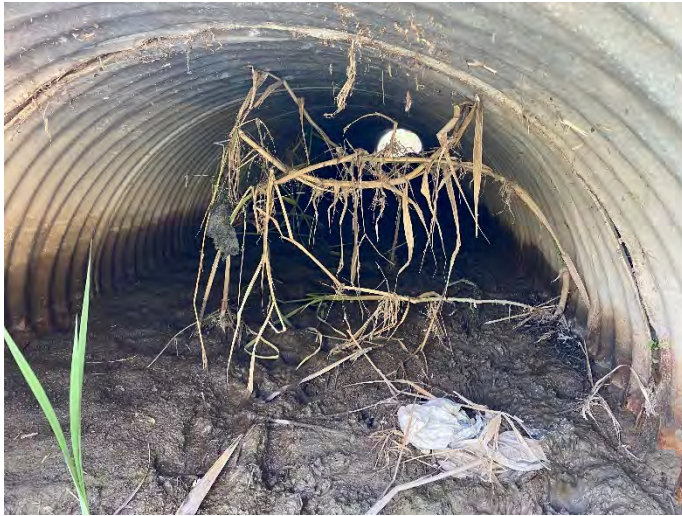
Photo 171: SC 11 – Downstream facing upstream inside culvert.
