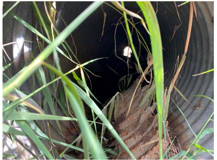
Photo 180: SC 12 – Upstream facing downstream inside culvert.
