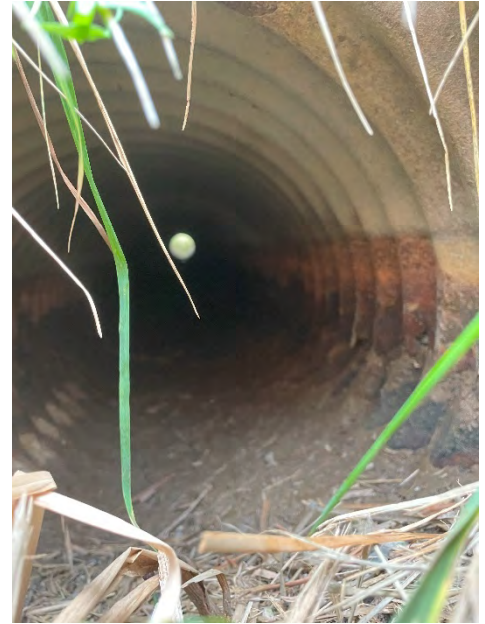
Photo 62: HC 1 – Downstream facing upstream inside culvert.
