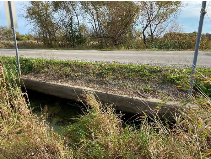
Photo 203: SC 22 – Upstream facing downstream towards culvert.
