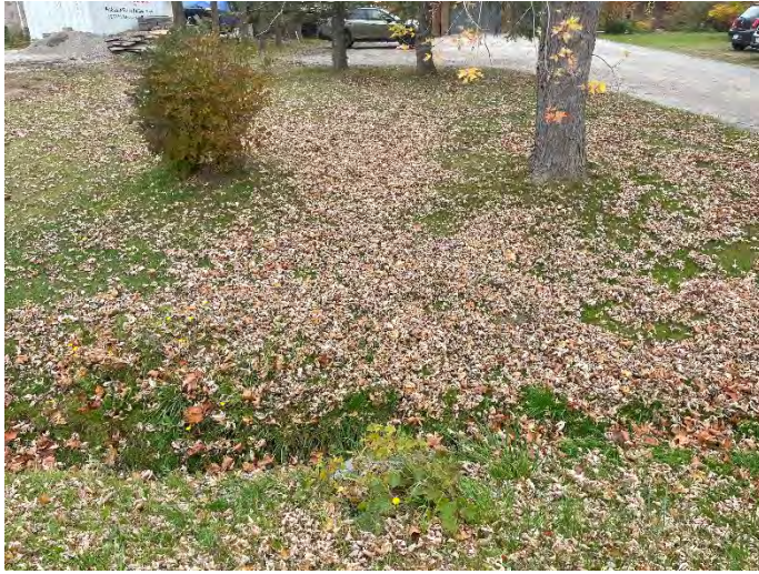
Photo 33: 20MC-W 4 – Facing upstream of culvert.
