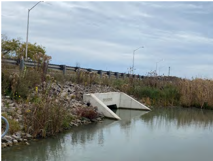
Photo 91: SHC 6 – Downstream facing upstream towards culvert.
