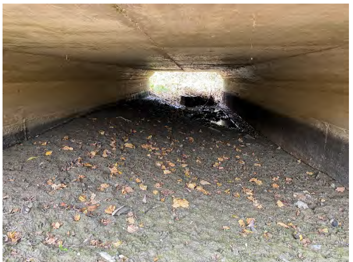
Photo 44: 20MC-E 9 – Downstream facing upstream inside culvert.
