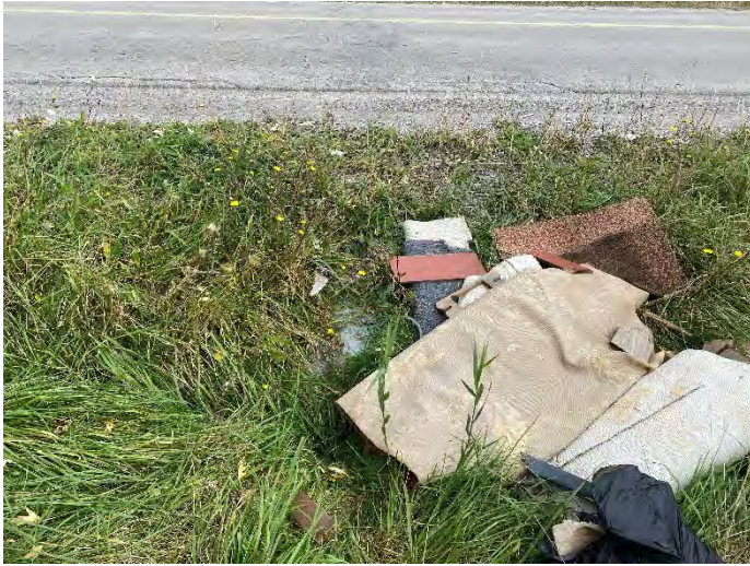
Photo 191: SC 18 – Upstream facing downstream towards culvert.
