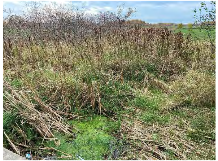
Photo 54: 20MC-W 13 – Facing downstream of culvert.
