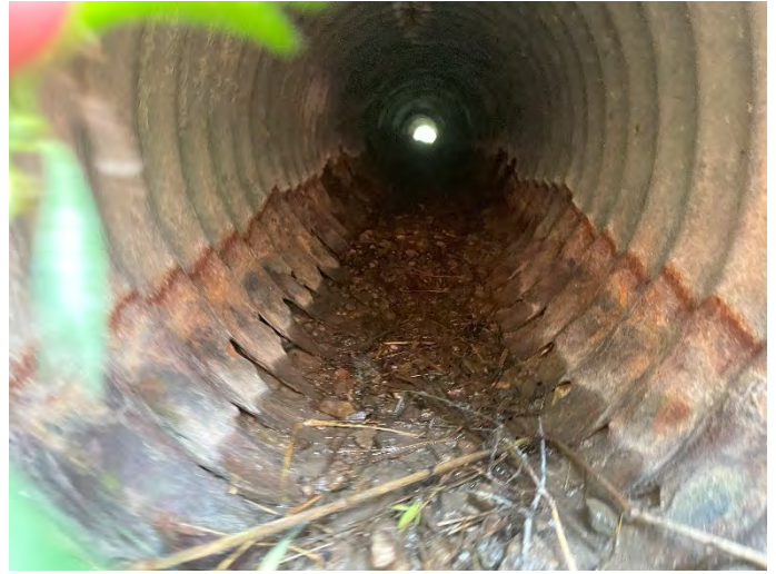
Photo 50: 20MC-E 15 – Downstream facing upstream inside culvert.
