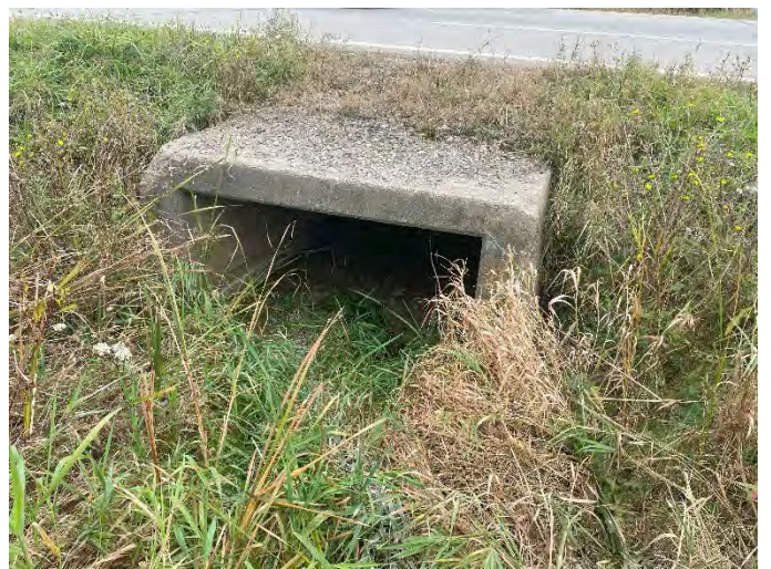
Photo 40: 20MC-E 3 – Upstream facing downstream towards culvert.
