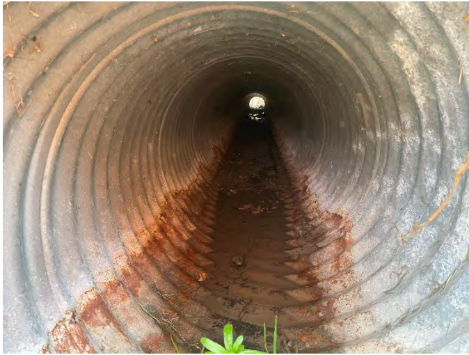
Photo 35: 20MC-W 4 – Upstream facing downstream inside culvert.
