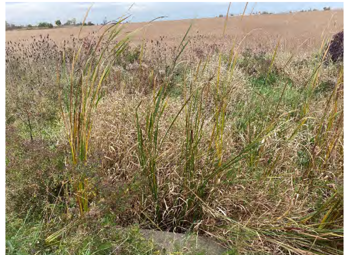
Photo 112: SHC 9 – Facing upstream of culvert.
