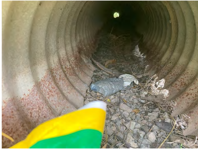
Photo 53: 20MC-E 15 – Upstream facing downstream inside culvert.
