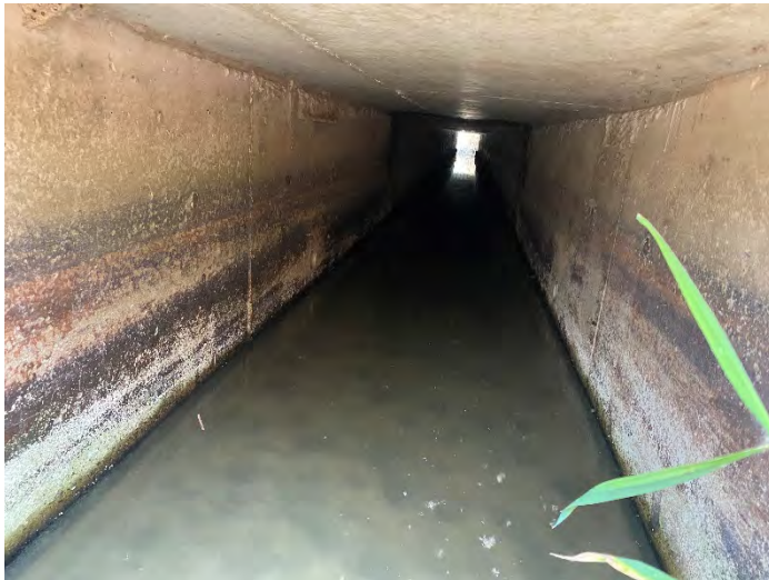
Photo 111: SHC 9 – Downstream facing upstream inside culvert.
