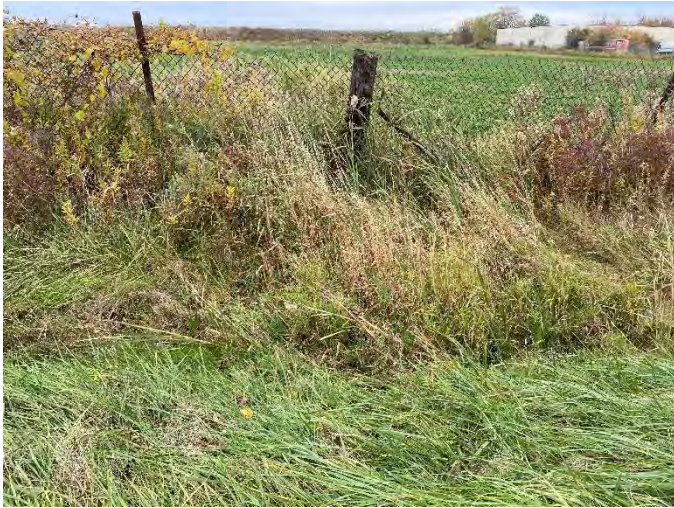
Photo 127: SHC 16 – Facing downstream of culvert.
