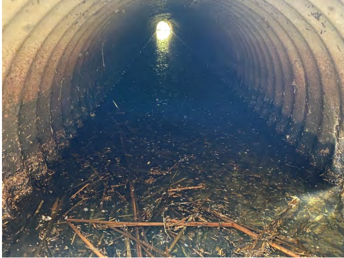
Photo 153: SC 8 – Downstream facing upstream inside culvert.
