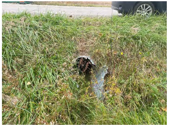
Photo 28: 20MC-W 3 – Upstream facing downstream towards culvert.
