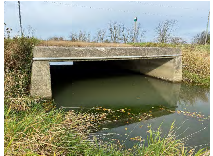
Photo 140: SHC 14 – Downstream facing upstream towards culvert.
