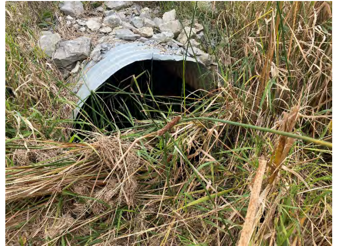
Photo 116: SHC 10 – Downstream facing upstream towards culvert.
