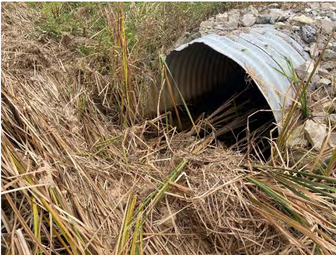
Photo 119: SHC 10 – Upstream facing downstream towards culvert.
