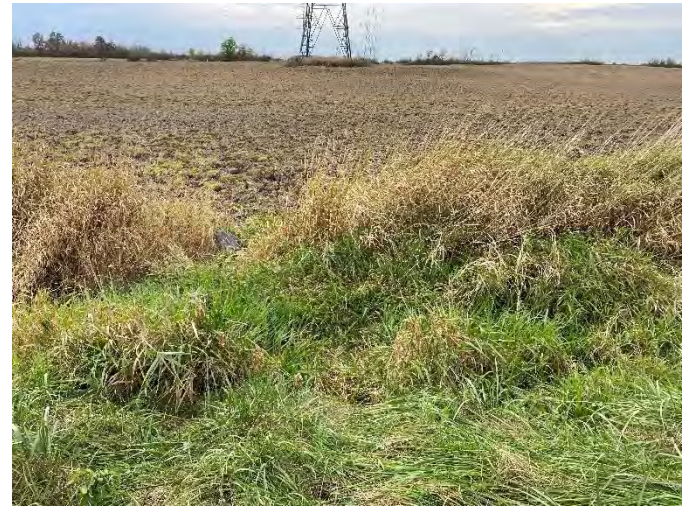
Photo 136: SHC 13 – Facing upstream of culvert.
