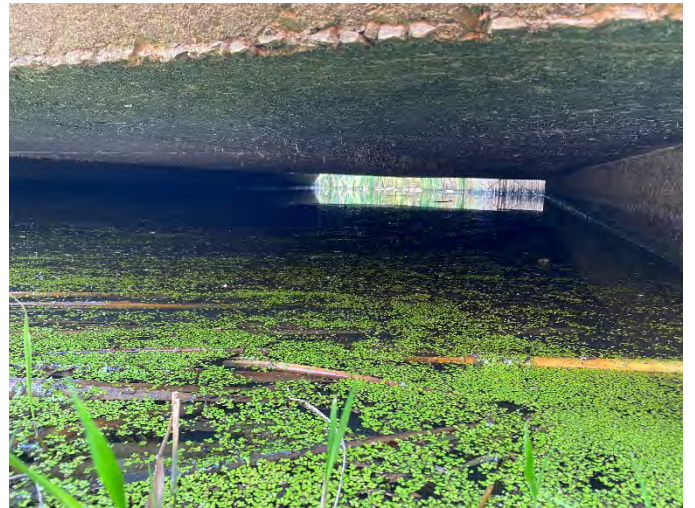
Photo 204: SC 22 – Upstream facing downstream inside culvert.
