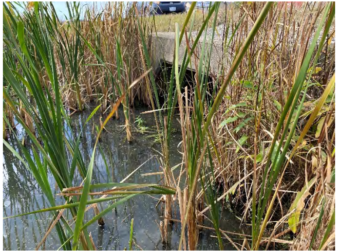
Photo 164: SC 2 – Downstream facing upstream towards culvert.
