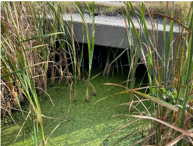
Photo 167: SC 2 – Upstream facing downstream towards culvert.
