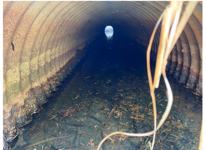
Photo 156: SC 8 – Upstream facing downstream inside culvert.
