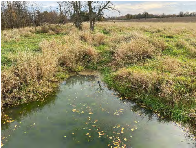
Photo 139: SHC 14 – Facing downstream of culvert.
