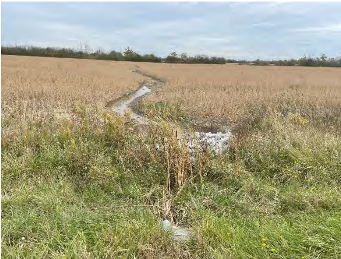
Photo 71: SHC 2 – Facing downstream of culvert.
