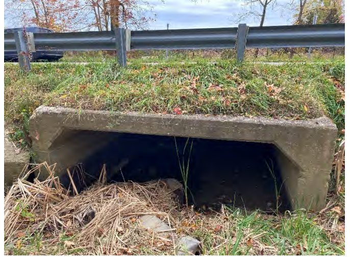
Photo 46: 20MC-E 9 – Upstream facing downstream towards culvert.
