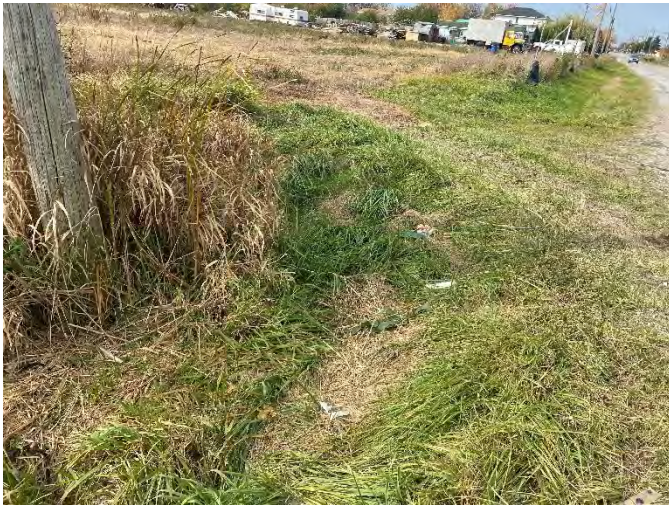
Photo 183: SC 23 – Upstream of culvert facing west.
