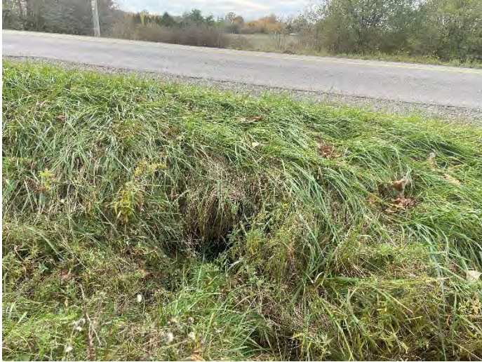
Photo 49: 20MC-E 15 – Downstream facing upstream towards culvert.
