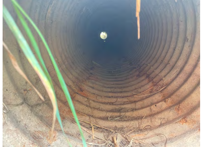
Photo 14: 20MC-W 1 – Downstream facing upstream inside culvert.
