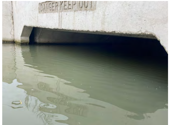
Photo 96: SHC 6 – Upstream facing downstream inside culvert.
