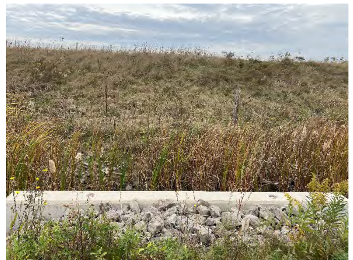
Photo 100: SHC 7 – Facing upstream of culvert.
