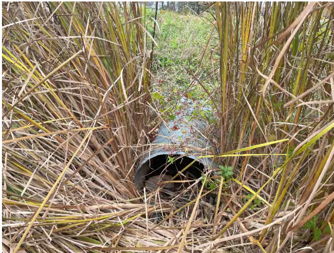
Photo 31: 20MC-W 4 – Downstream facing Upstream towards culvert.
