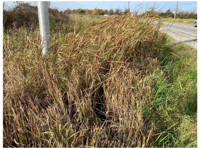
Photo 160: SC 5 – Facing upstream of culvert.
