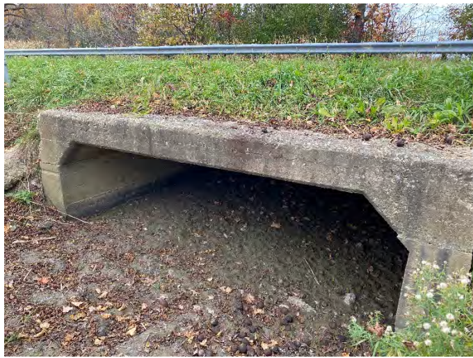
Photo 43: 20MC-E 9 – Downstream facing upstream towards culvert.
