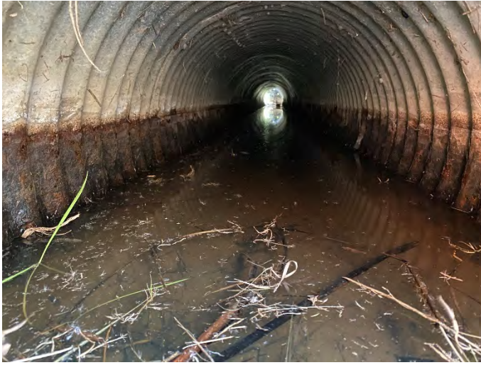
Photo 123: SHC 15 – Downstream facing upstream inside culvert.
