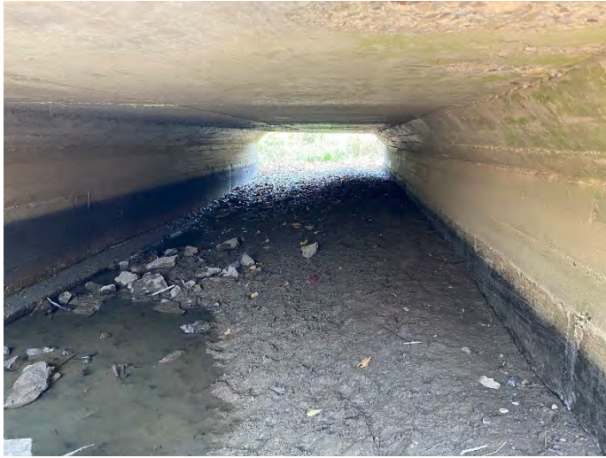
Photo 47: 20MC-E 9 – Upstream facing downstream inside culvert.
