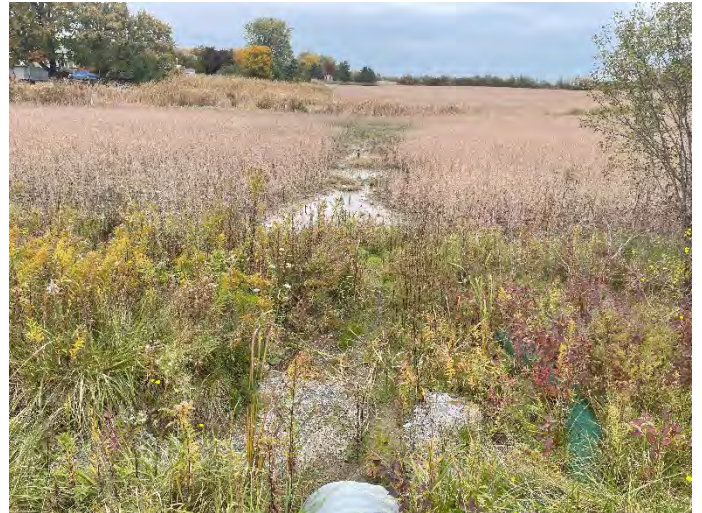
Photo 24: 20MC-W 3 – Facing downstream of culvert.
