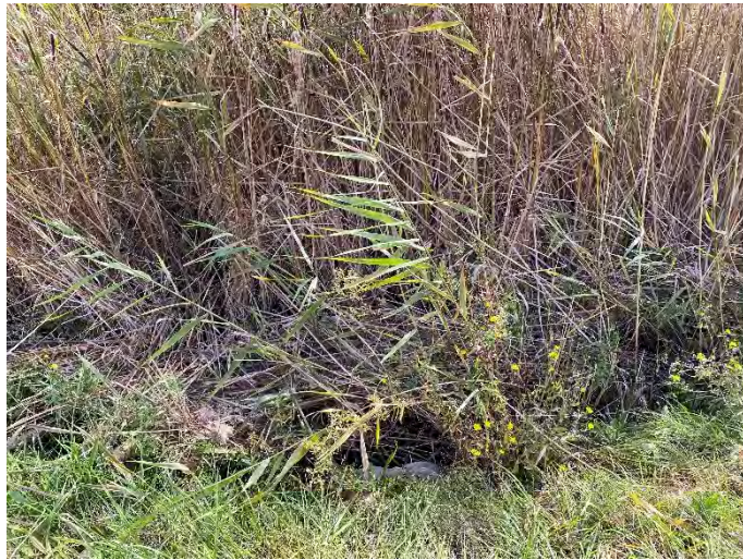
Photo 151: SC 8 – Facing downstream of culvert.
