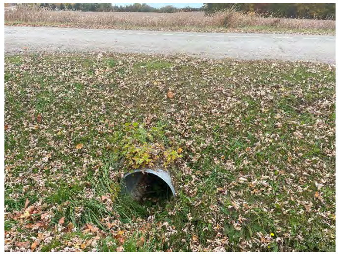
Photo 34: 20MC-W 4 – Upstream facing downstream towards culvert.
