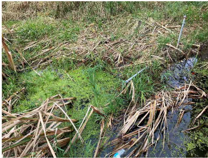
Photo 57: 20MC-W 13 – Facing upstream of culvert.
