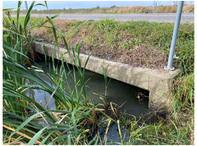
Photo 200: SC 22 – Downstream facing upstream towards culvert.
