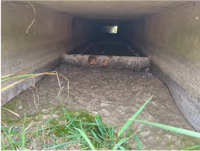
Photo 41: 20MC-E 3 – Upstream facing downstream inside culvert.
