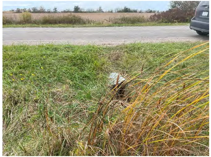
Photo 72: SHC 2 – Downstream facing upstream towards culvert.
