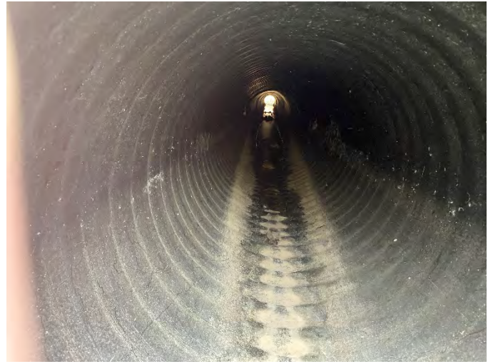
Photo 108: SHC 8 – Upstream facing downstream inside culvert.
