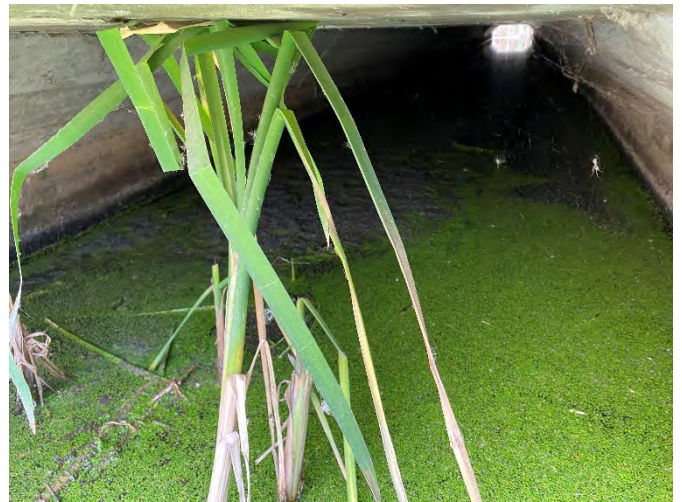
Photo 168: SC 2 – Upstream facing downstream inside culvert.
