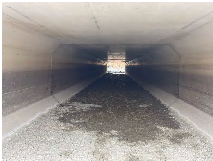
Photo 88: SHC 5 – Upstream facing downstream inside culvert.
