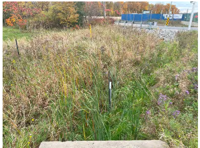
Photo 36: 20MC-E 3 – Facing downstream of culvert.
