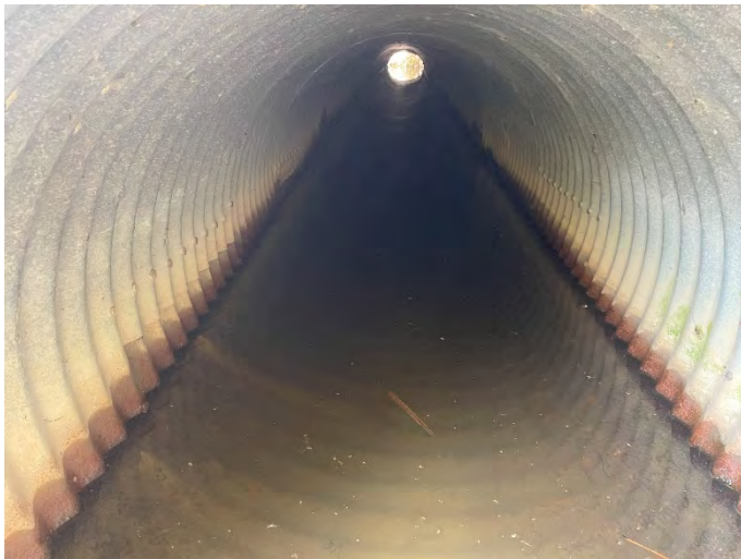
Photo 23: 20MC-W 2 – Upstream facing downstream inside culvert.
