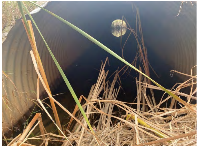
Photo 120: SHC 10 – Upstream facing downstream inside culvert.
