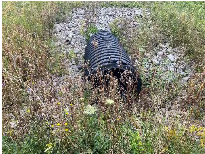
Photo 107: SHC 8 – Upstream facing downstream towards culvert.
