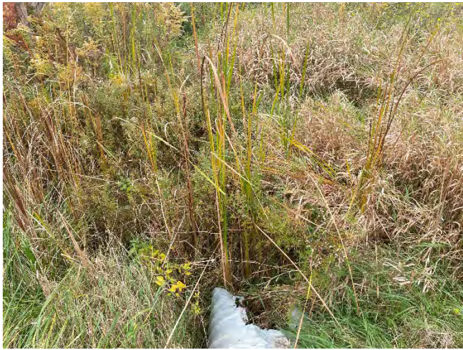
Photo 15: 20MC-W 1 – Facing upstream of culvert.
