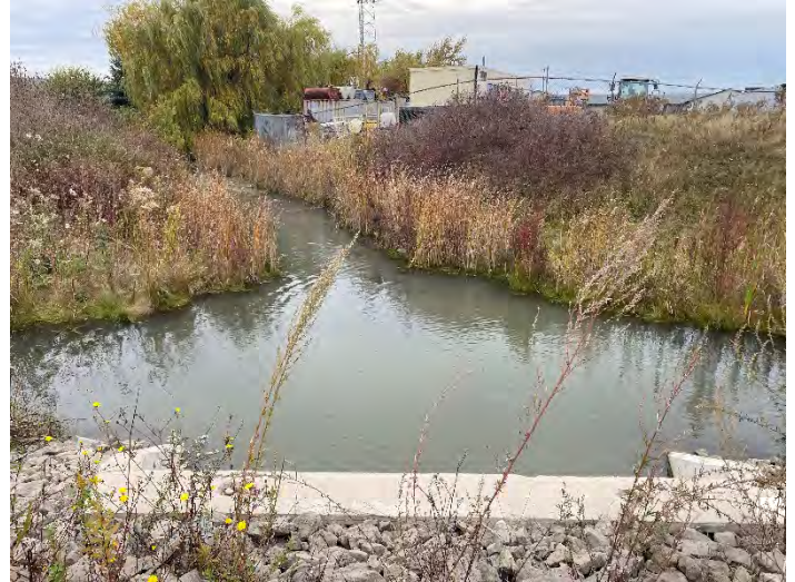
Photo 94: SHC 6 – Facing upstream of culvert.
