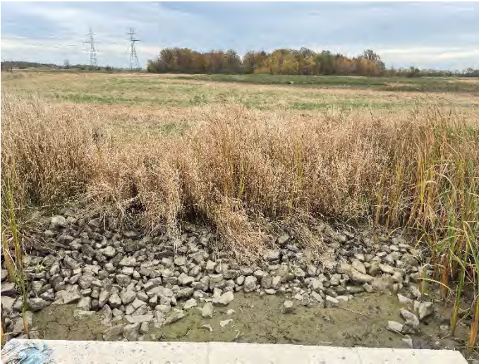
Photo 83: SHC 5 – Facing downstream of culvert.
