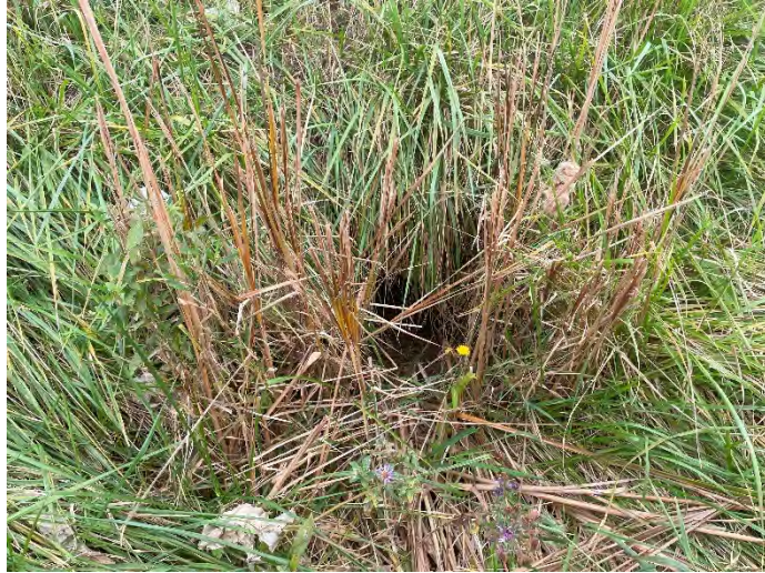
Photo 61: HC 1 – Downstream facing upstream towards culvert.
