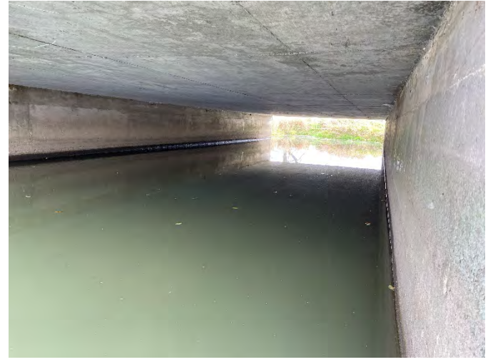
Photo 144: SHC 14 – Upstream facing downstream inside culvert.
