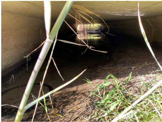
Photo 159: SC 5 – Downstream facing upstream inside culvert.
