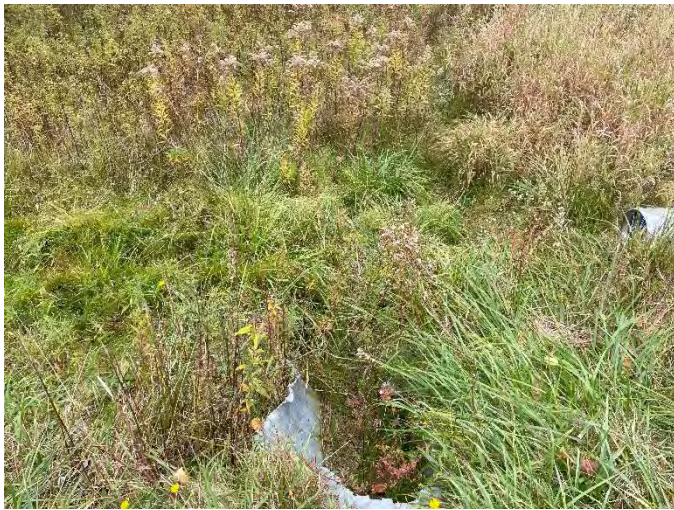
Photo 27: 20MC-W 3 – Facing upstream of culvert.
