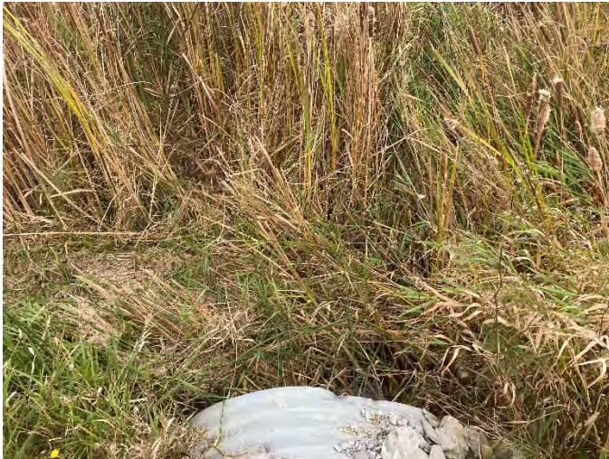
Photo 115: SHC 10 – Facing downstream of culvert.
