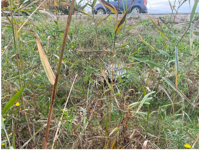
Photo 13: 20MC-W 1 – Downstream facing upstream towards culvert.
