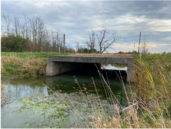
Photo 143: SHC 14 – Upstream facing downstream towards culvert.
