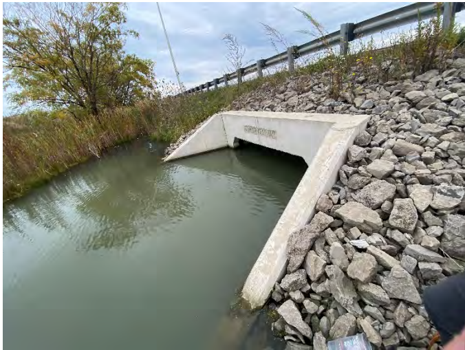
Photo 95: SHC 6 – Upstream facing downstream towards culvert.
