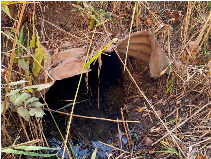
Photo 155: SC 8 – Upstream facing downstream towards culvert.
