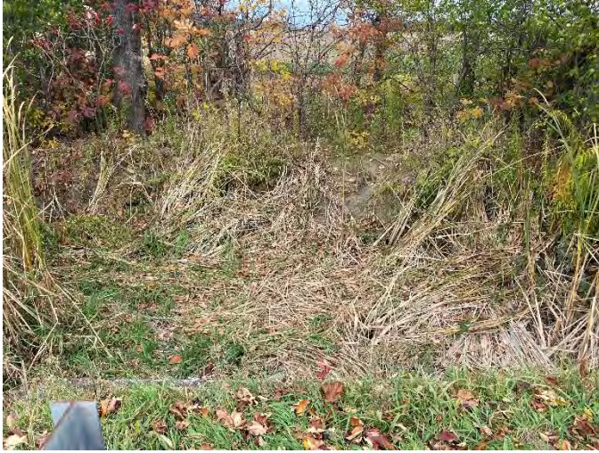
Photo 45: 20MC-E 9 – Facing upstream of culvert.
