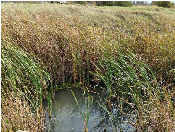
Photo 163: SC 2 – Facing downstream of culvert.
