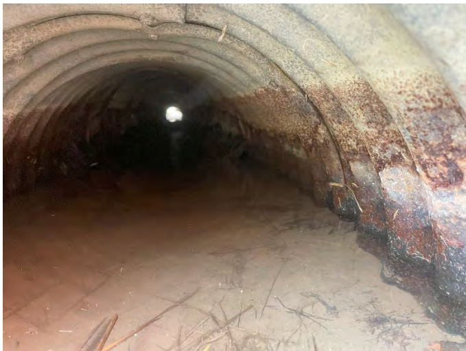
Photo 11: 20MC-W 12 – Upstream facing downstream inside culvert.
