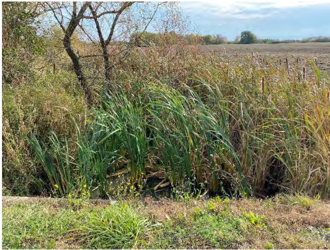
Photo 199: SC 22 – Facing downstream of culvert.
