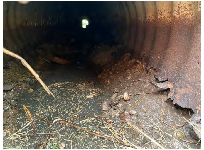
Photo 132: SHC 16 – Upstream facing downstream inside culvert.
