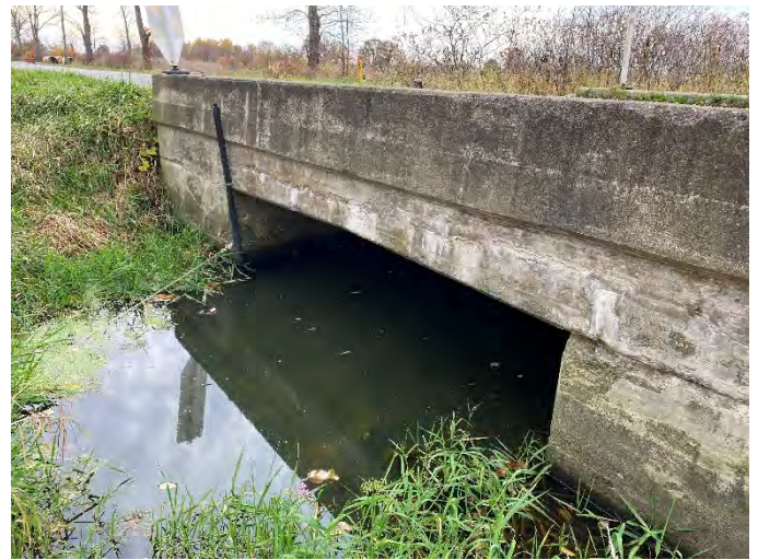
Photo 58: 20MC-W 13 – Upstream facing downstream towards culvert.
