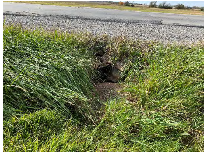
Photo 148: SC 7 – Upstream facing downstream towards culvert.
