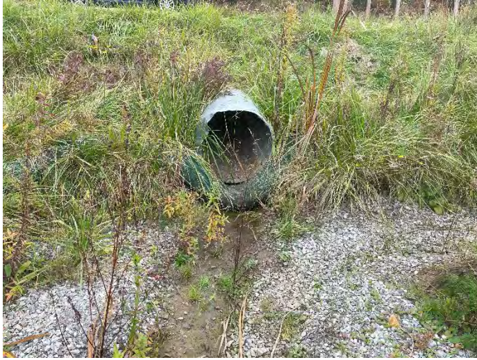
Photo 25: 20MC-W 3 – Downstream facing upstream towards culvert.
