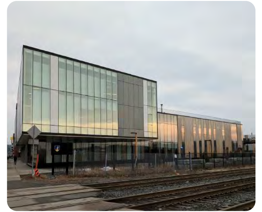
Institutional Building Precedent - Sudbury, ON
