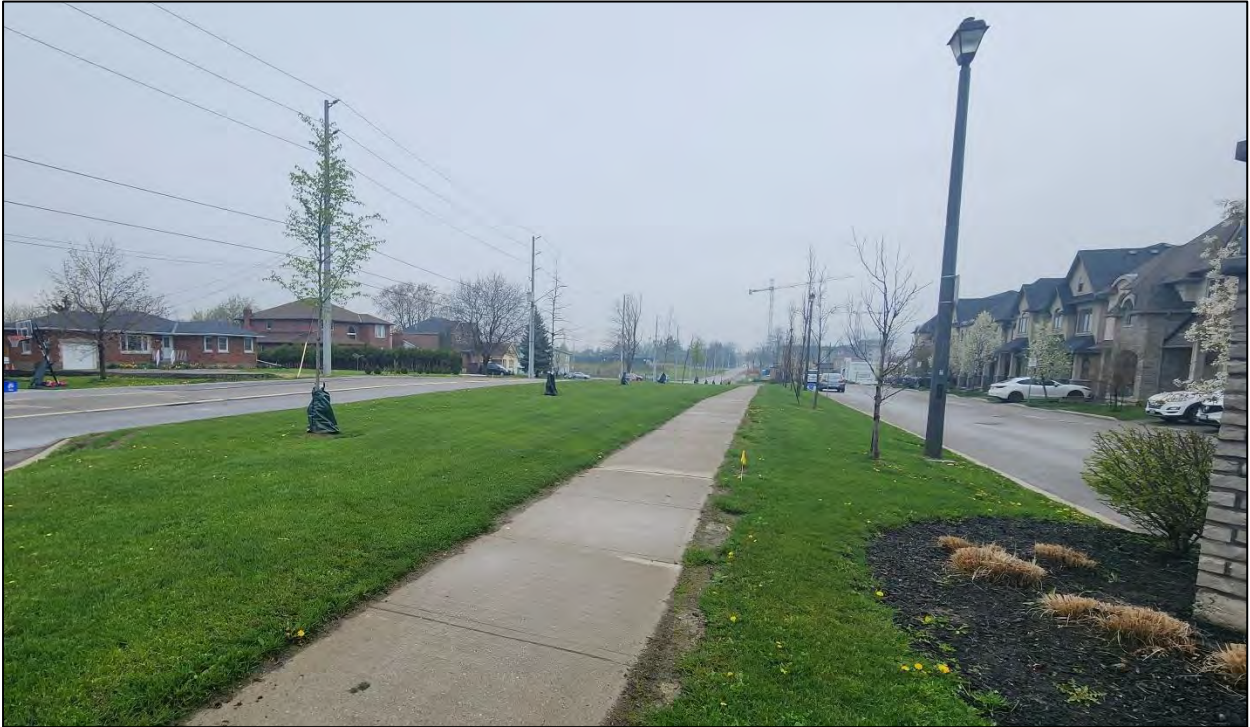
Figure 2.4) West 5 th Street Sidewalk Condition – 1137-1175 West 5 th Street
