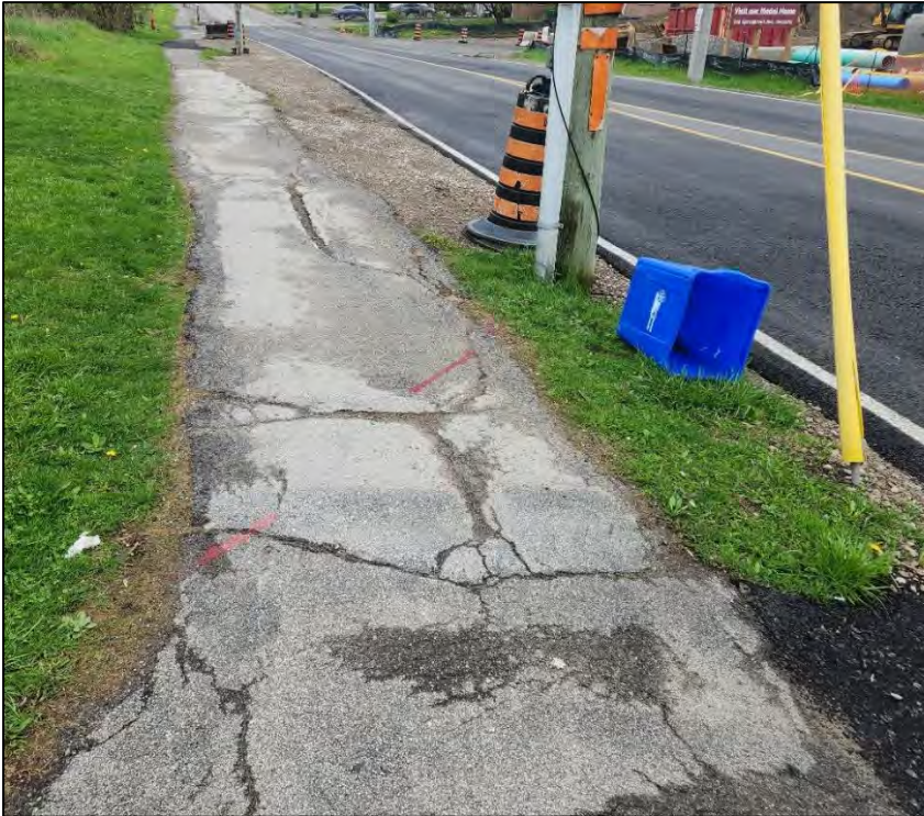
Figure 2.3) West 5th Street Sidewalk Condition – Heavy Vehicle Damage
