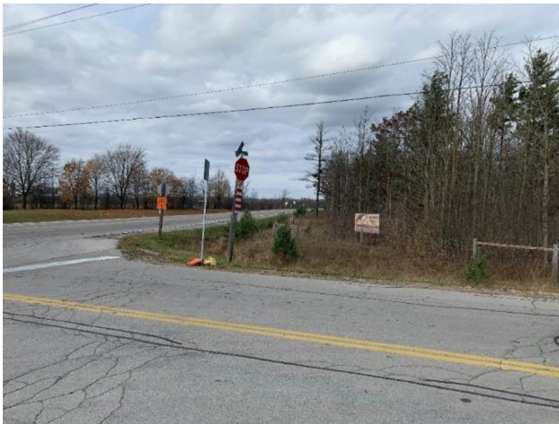
Image 2: Safari Road and Kirkwell Road intersection. Test pit survey required beyond disturbed, elevated roadbed.
