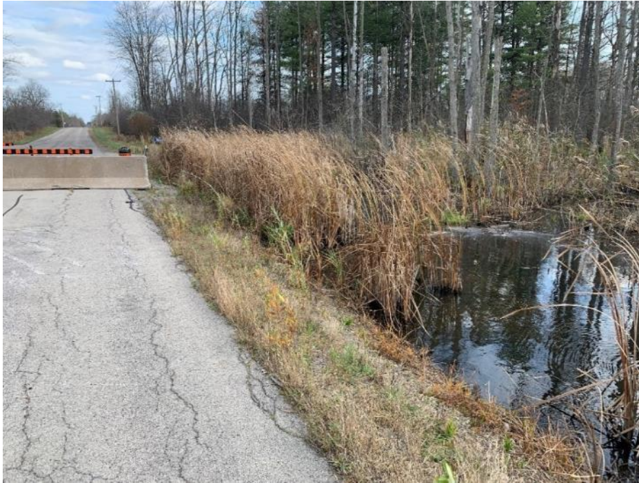
Image 15: Low and wet conditions beyond Safari Road within the Provincially Significant Wetland. Low archaeological potential.
