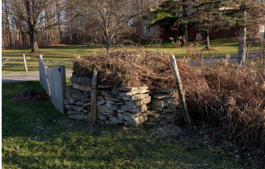
Figure 3.5 Close up of Stone Landscape Feature at 1267 Valens Road
