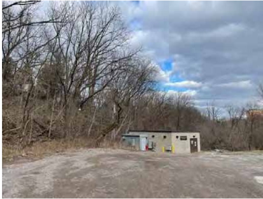
Photo 1: HD011 Pumping station at Alternative Site 1
