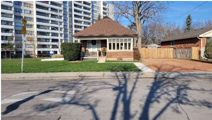
Plate 4: South elevation of the residence at 88 Ofield Road in the location of Site 4, looking north from Ofield Road (A.S.I. 2022).
