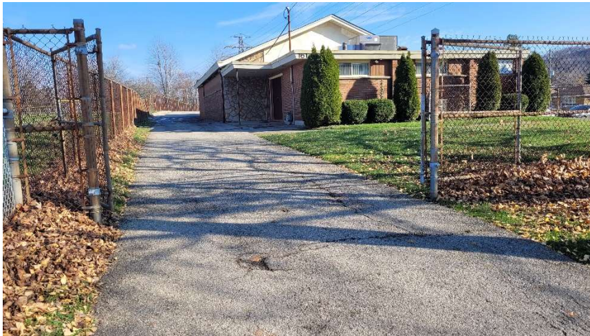
Plate 13: Church and entrance driveway at Site 19 – 161 Rifle Range Road, looking east from Rifle Range Road (A.S.I. 2022).
