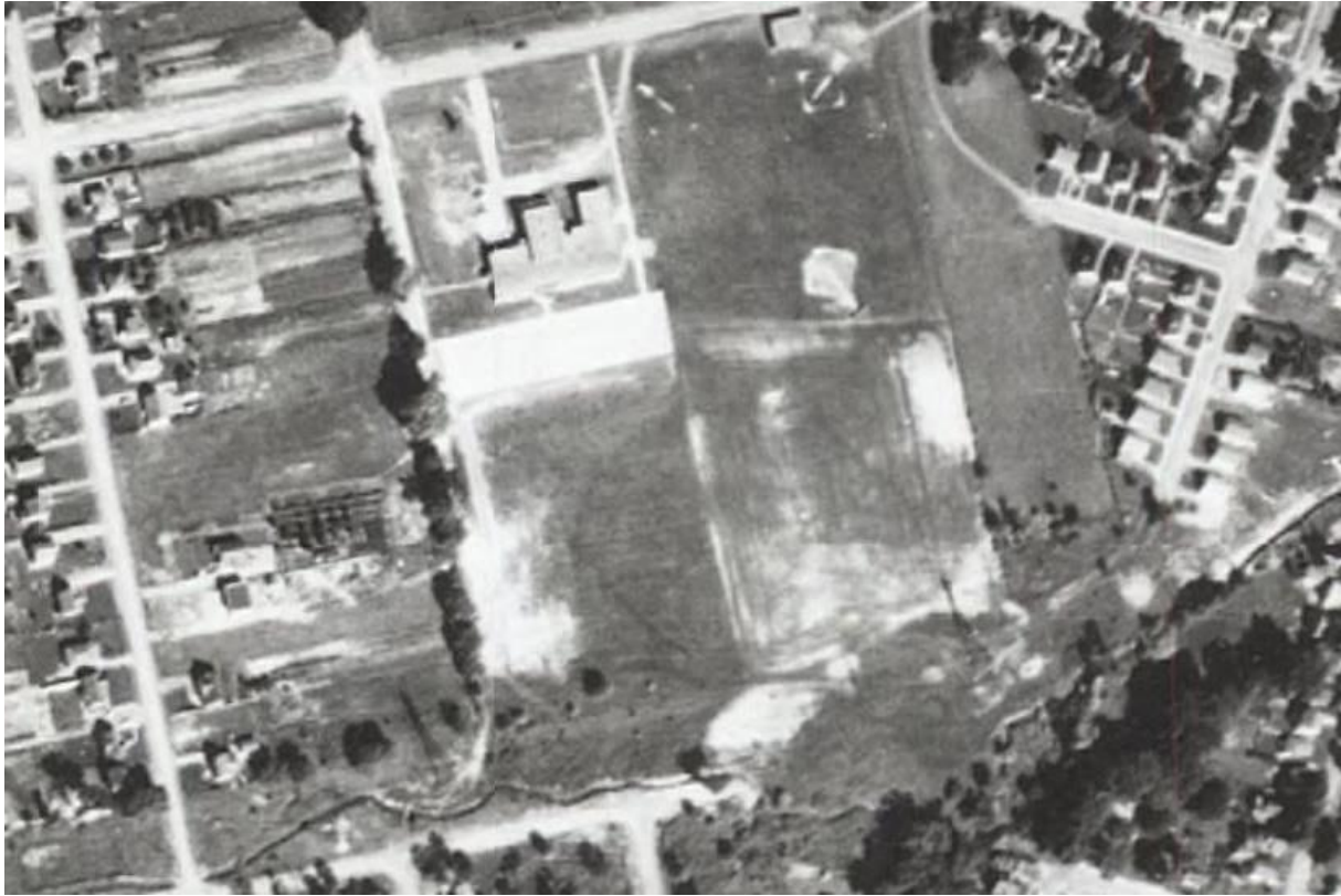
Image 17: Sites 12 and 19 area showing the lands being cleared prior to construction of the extant building at Site 19.
