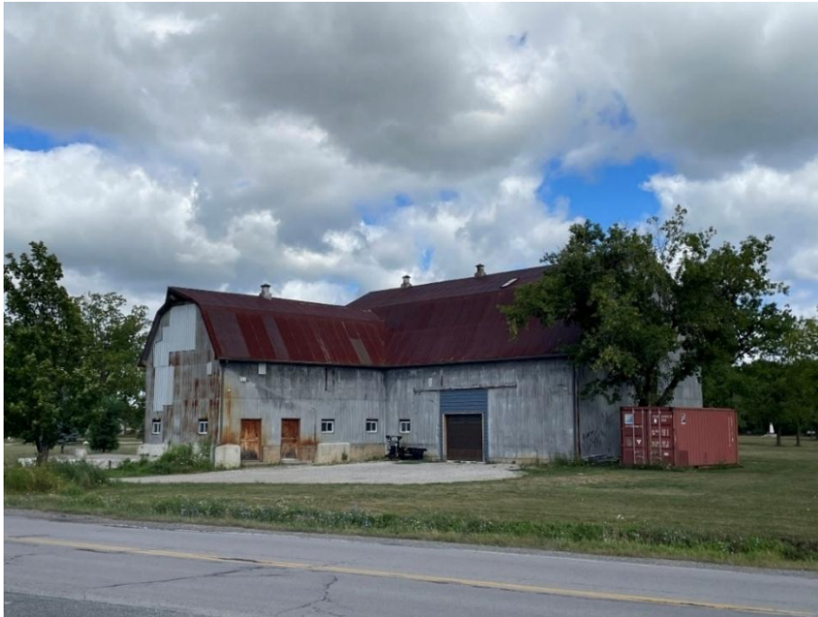
Plate 7: Facade of B.H.R. 1, taken from opposite side of White Church Road looking north (A.S.I. 2025).
