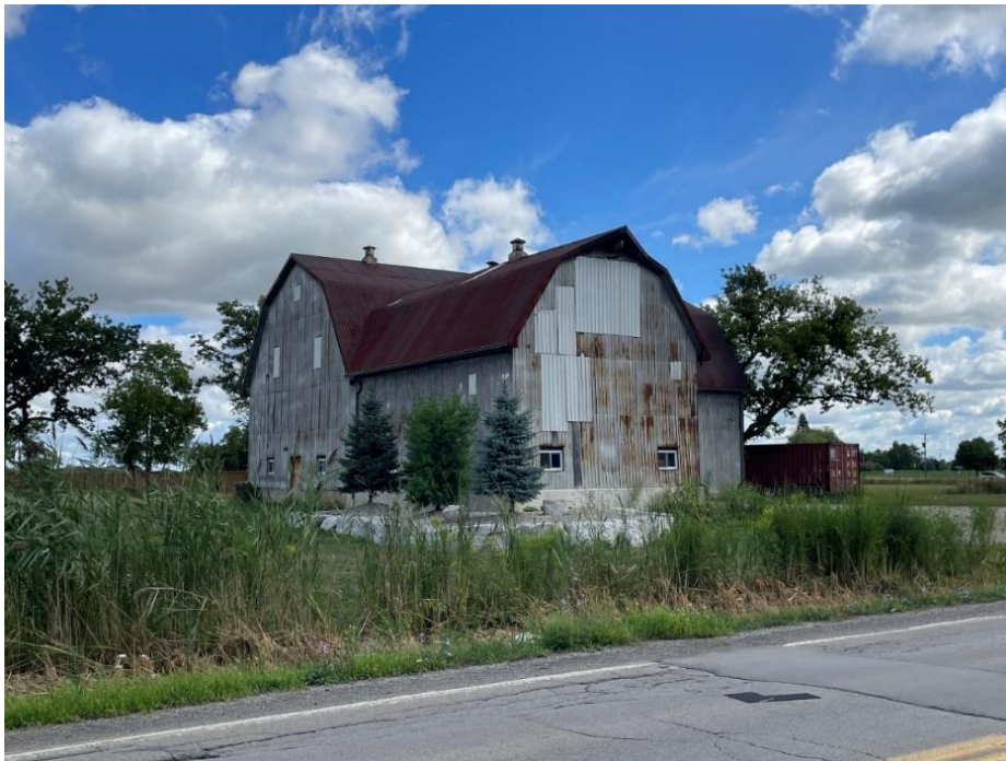
Plate 8: Western side of B.H.R. 1, taken from opposite side of White Church Road looking north (A.S.I. 2025).
