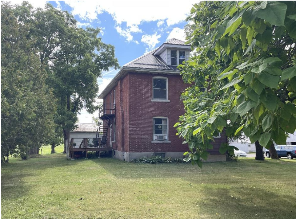
Plate 9: Residential structure at Potential C.H.L. 2, looking east (A.S.I. 2025).
