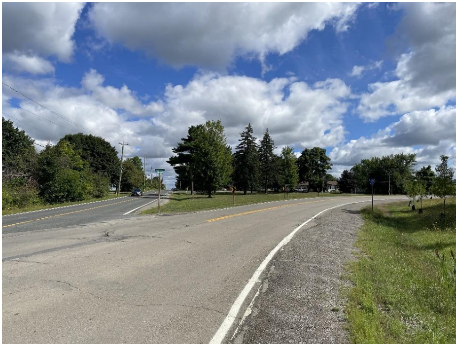
Plate 4: Taken from middle portion of Binbrook Intersection, looking north (A.S.I. 2025).
