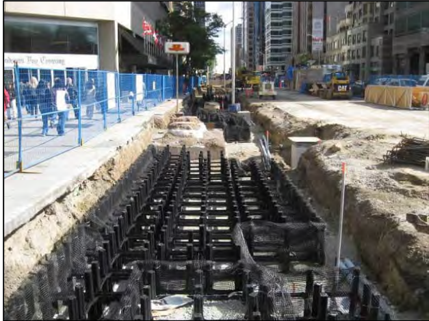
Figure 5-2: Tree Planter/Soil Retention Cell Construction ( www.smartcitiesdive.com , 2020)
