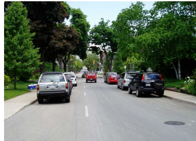
Bay Street After
