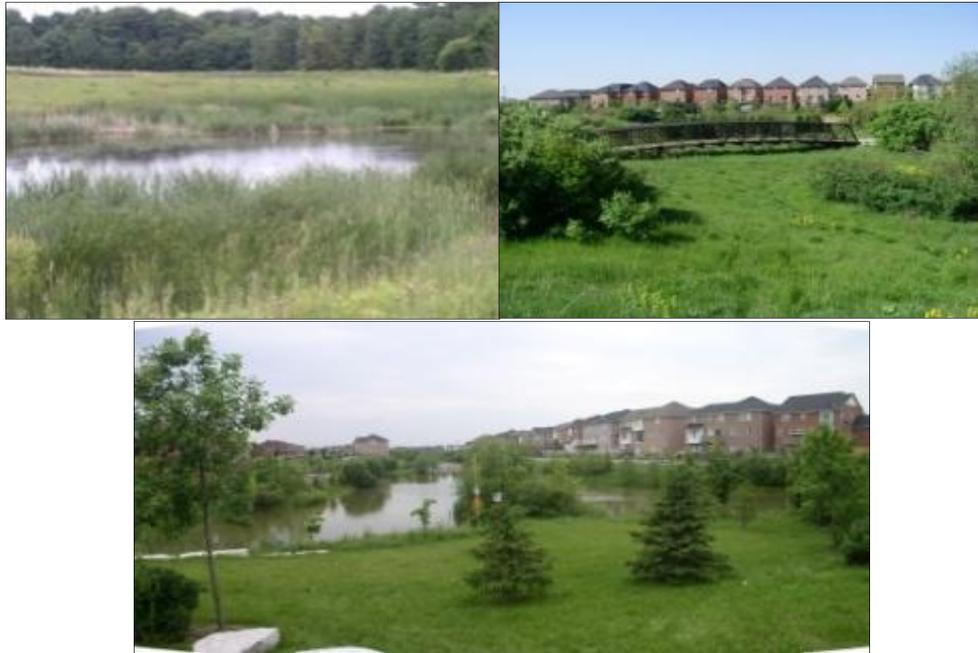
**Figure 7.8.1: Example End-of-Pipe Controls (clockwise from top left: Constructed Wetland, Dry Pond, Wet Pond)**
