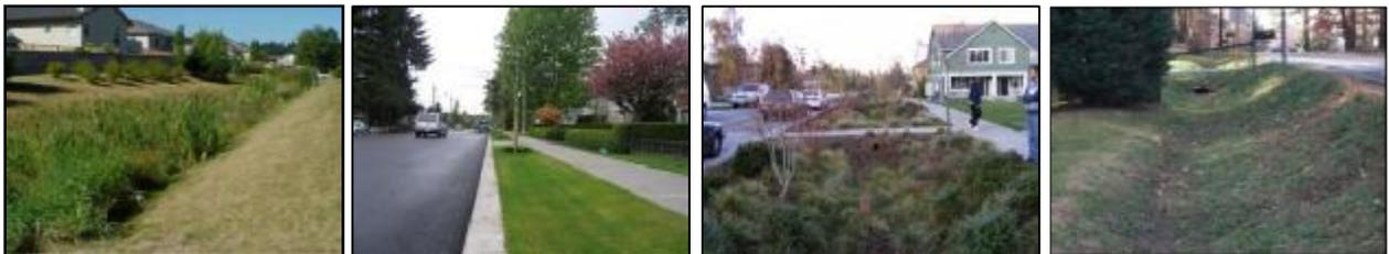
**Figure 7.8.4: Example LID Conveyance Controls (From L to R: Vegetated Channel, Subsurface Perforated Pipe, Bio-swale, Grass Channel)**
