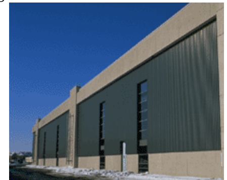
Solar Wall, Ford Plant in Oakville, ON
