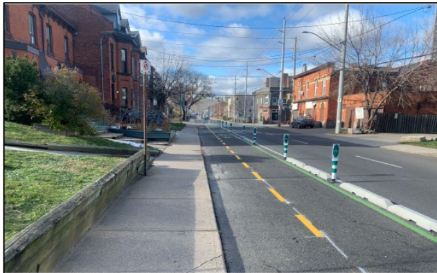
Hunter St, Hamilton Flexposts and pre-cast curbs.
